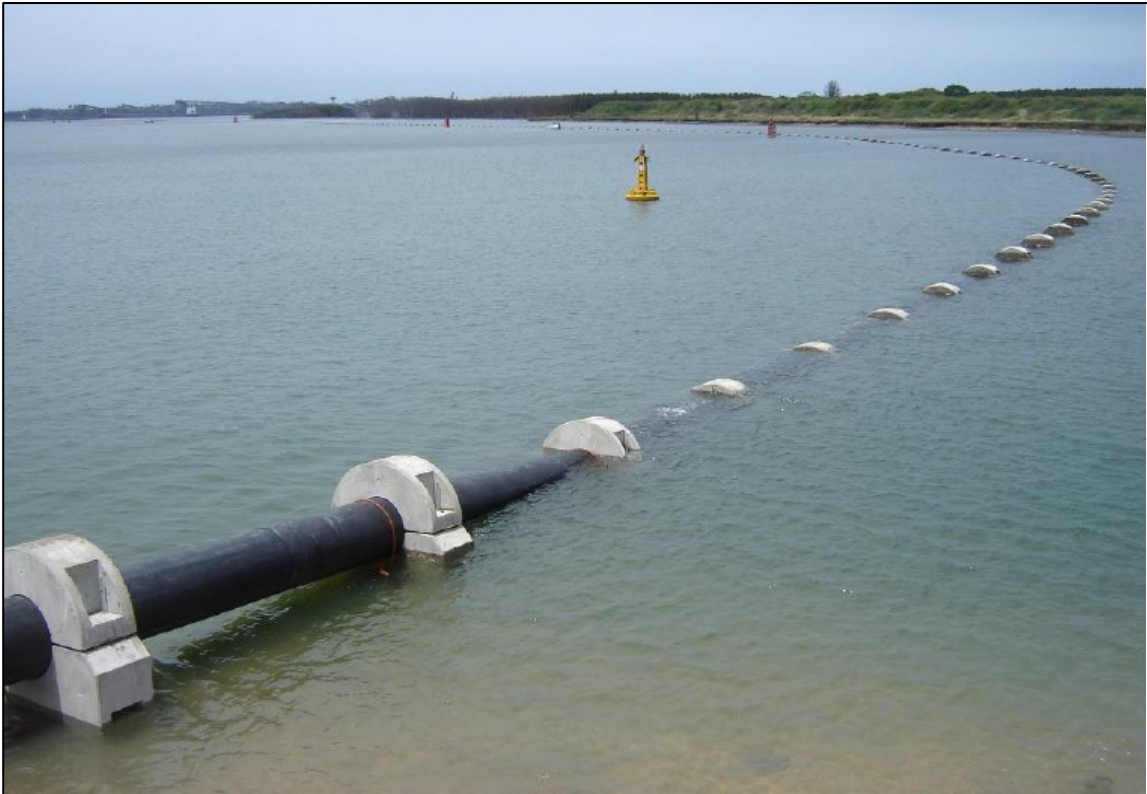
Plate 2.7: Example of HDPE pipeline with collars to provide hydrodynamic stability when placed on the seabed (WSP).
