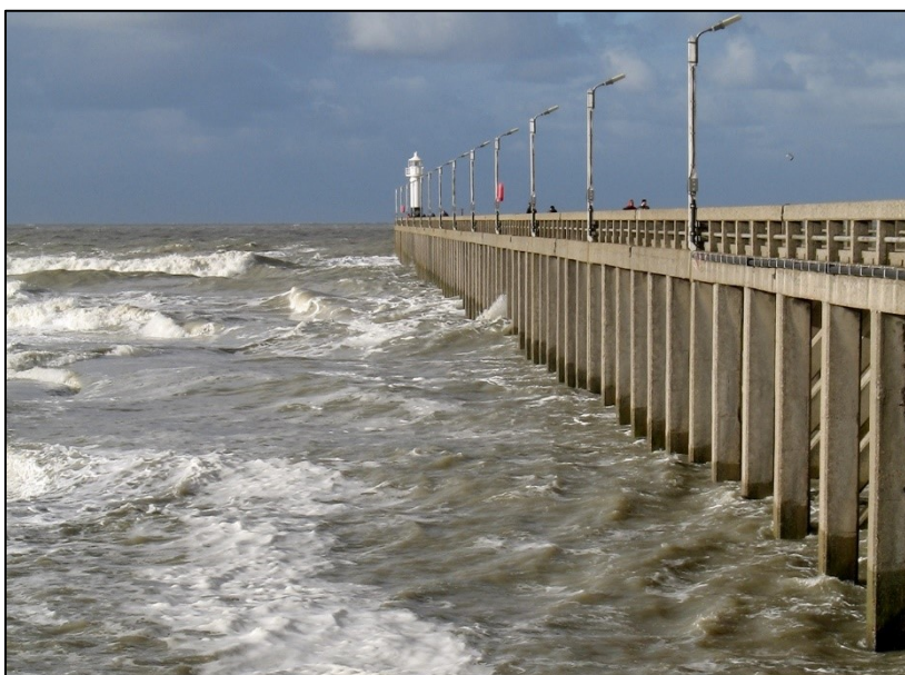
Plate 2.4: Example of intake jetty.
