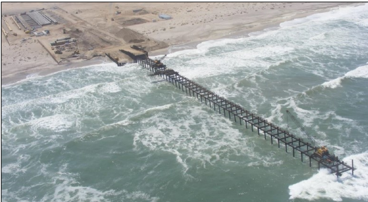
Figure 2.10: Sheet pile jetty structure to provide access for cranes to excavate pipe burial trench (WSP, 2020).
