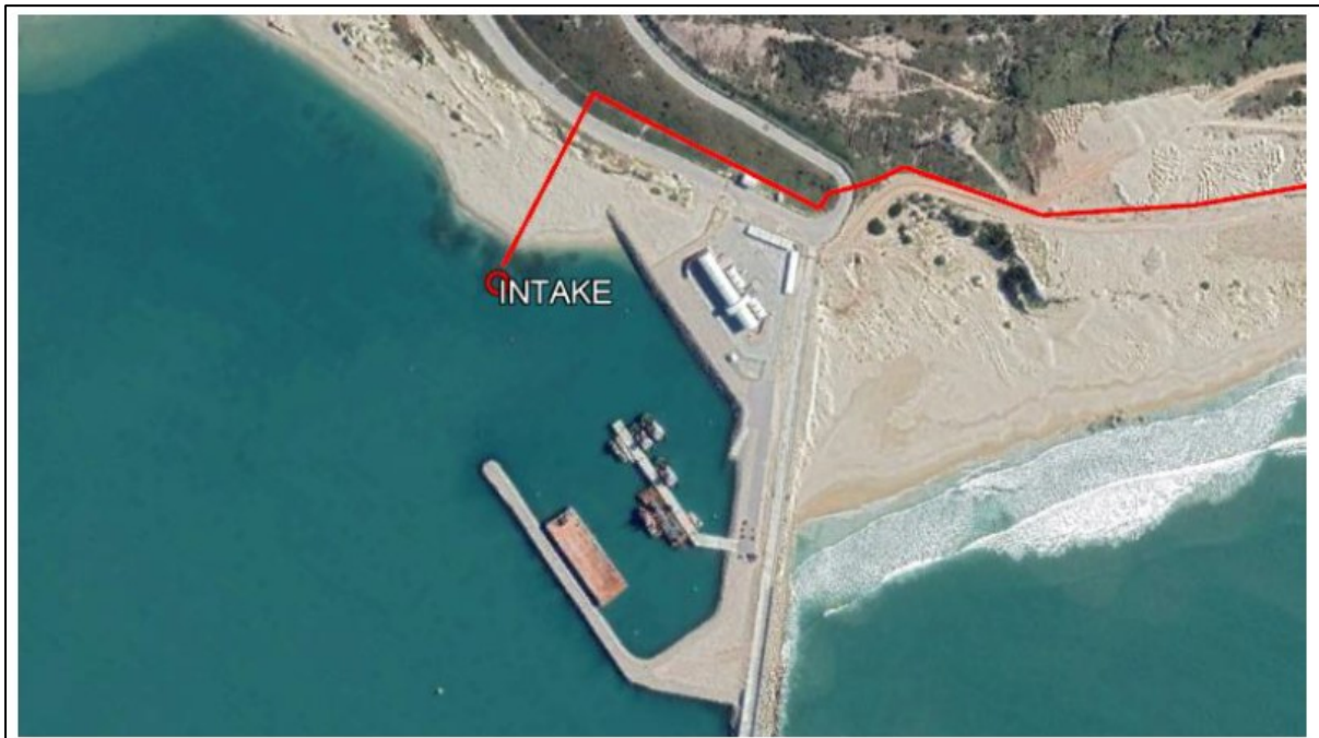
Plate 2.3: Intake for cooling water located within the Port of Ngqura (Source: WSP, 2020)
