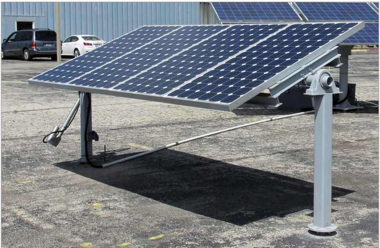
Figure 13: Example of PV Module mounted on Single Axis Tracker
