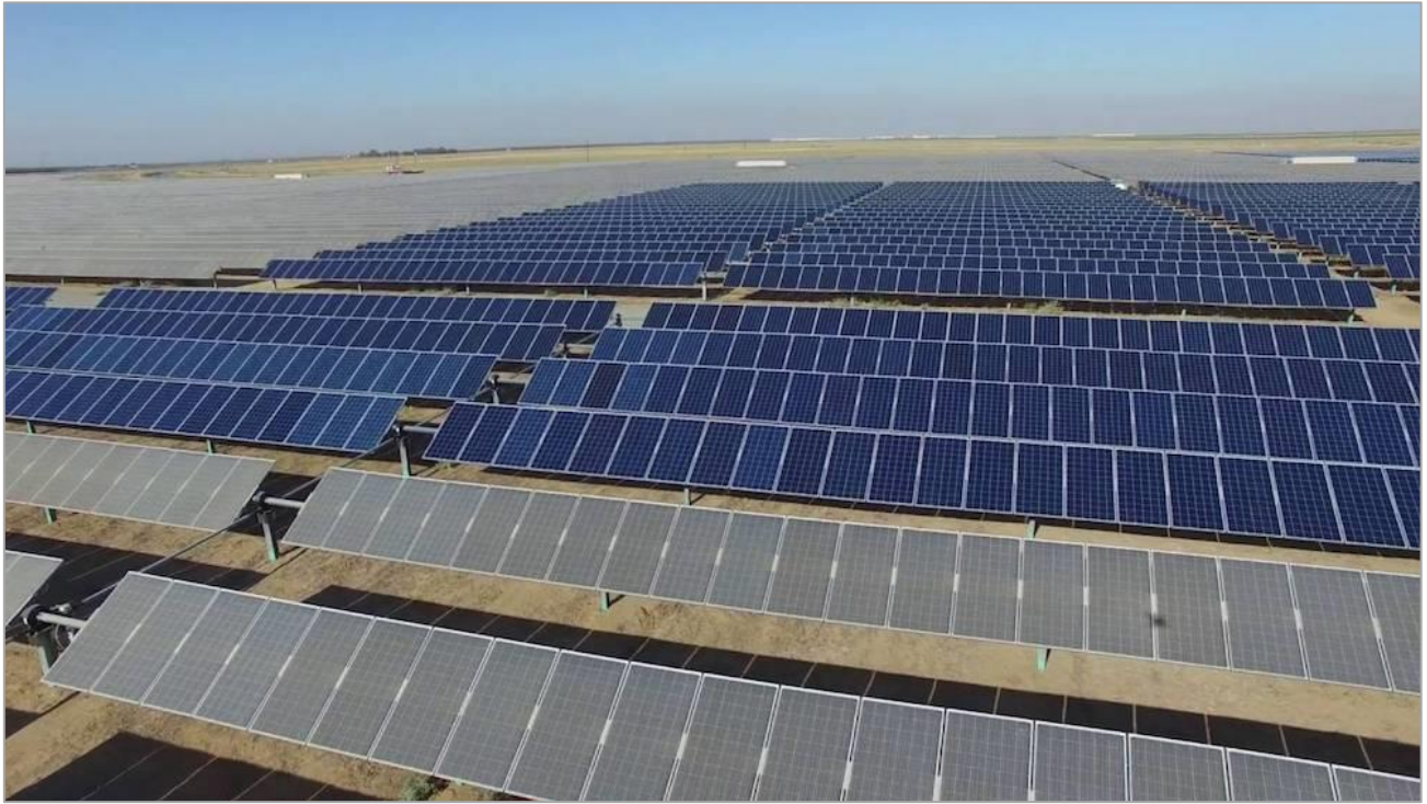
Figure 17: Example of Roads Between Trackers and Medium Voltage Substations (source: https://ecoinventos.com/ )
