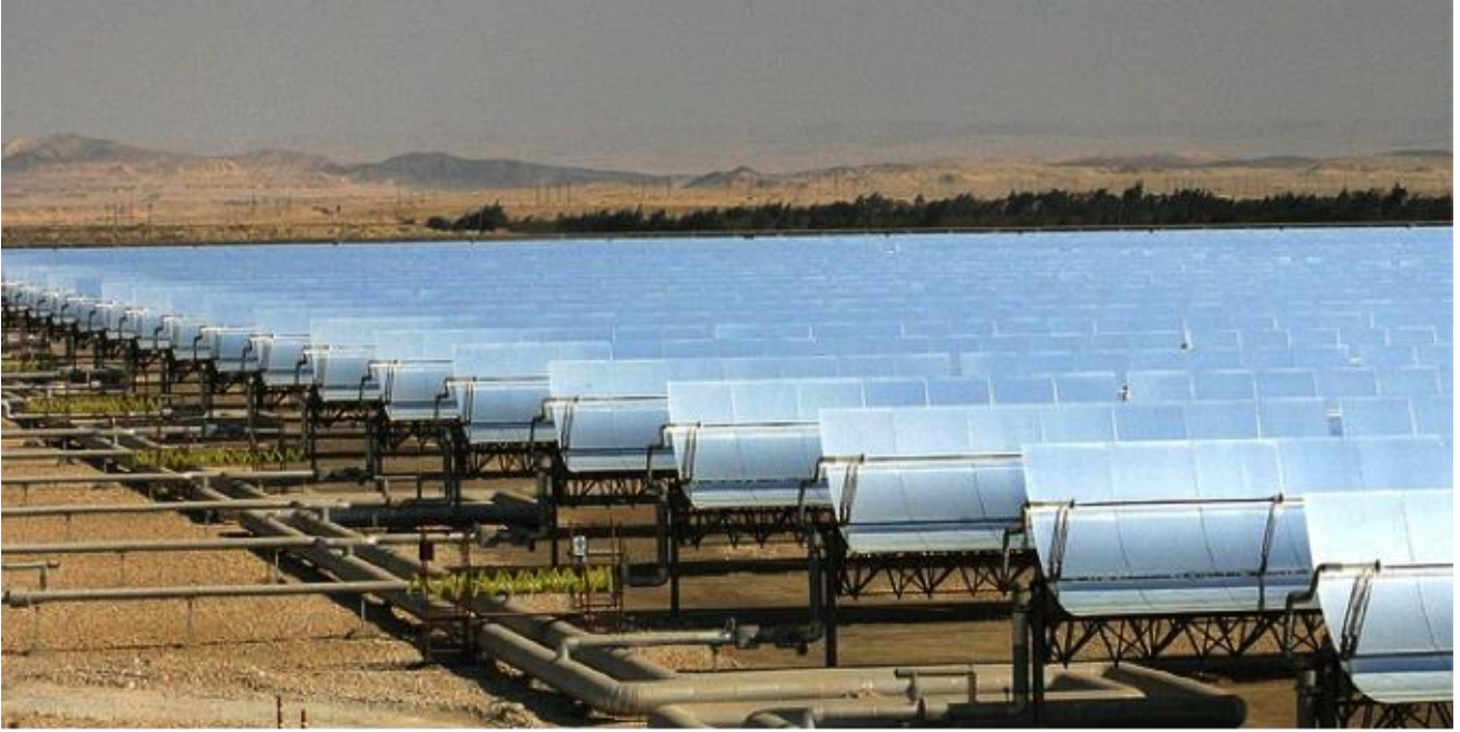
Figure 7: Parabolic Trough Technology ( www.e-education.psu.edu )
