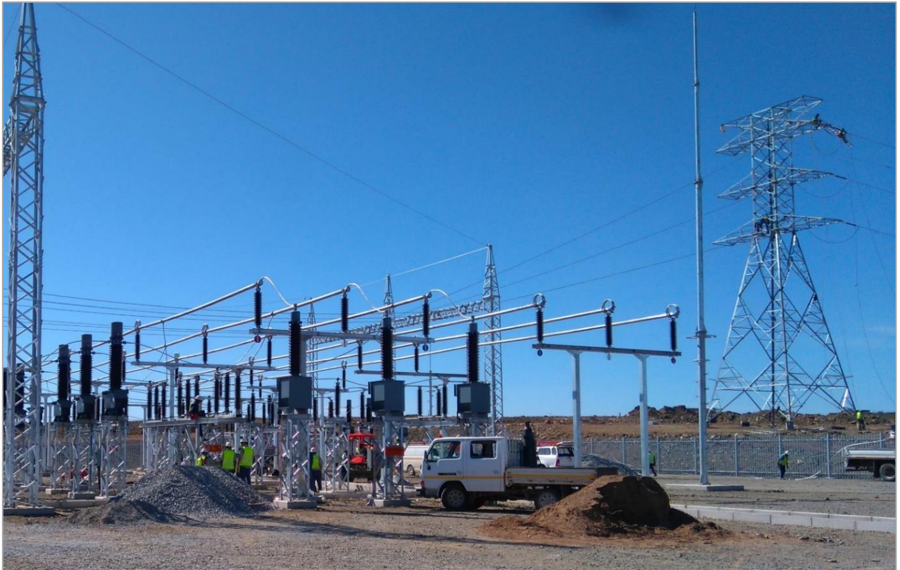
Figure 21: Example of High Voltage Transmission Line Connecting to Substation
