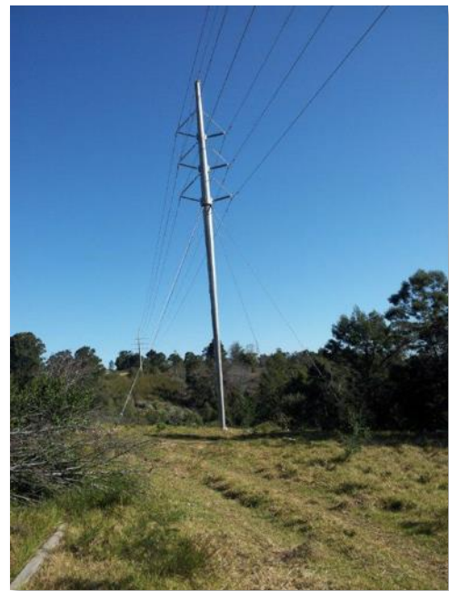
Figure 4-6: Example of a Guyed-suspension
