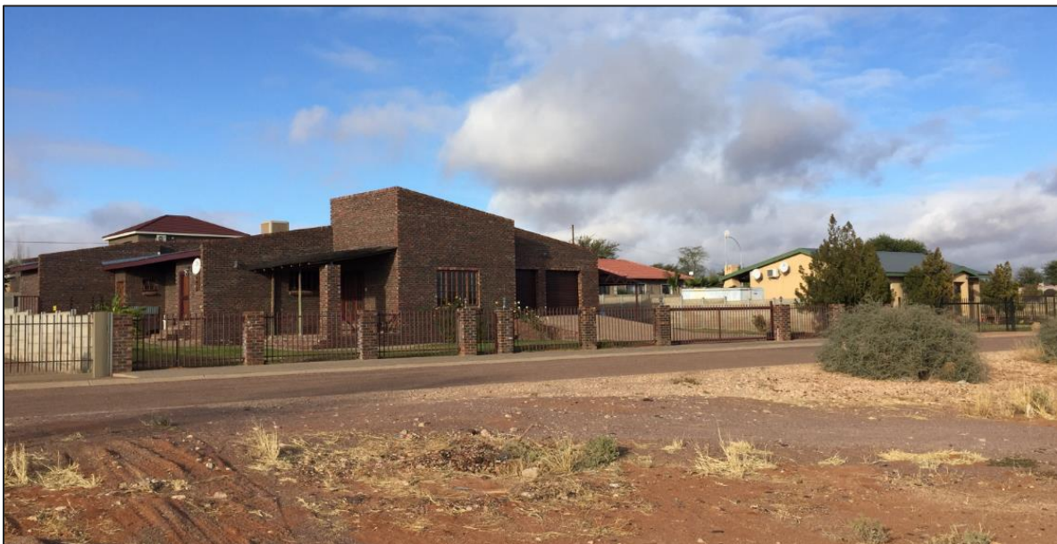
Figure 6-21: Photograph 9 depicting the Upington residential built environment
