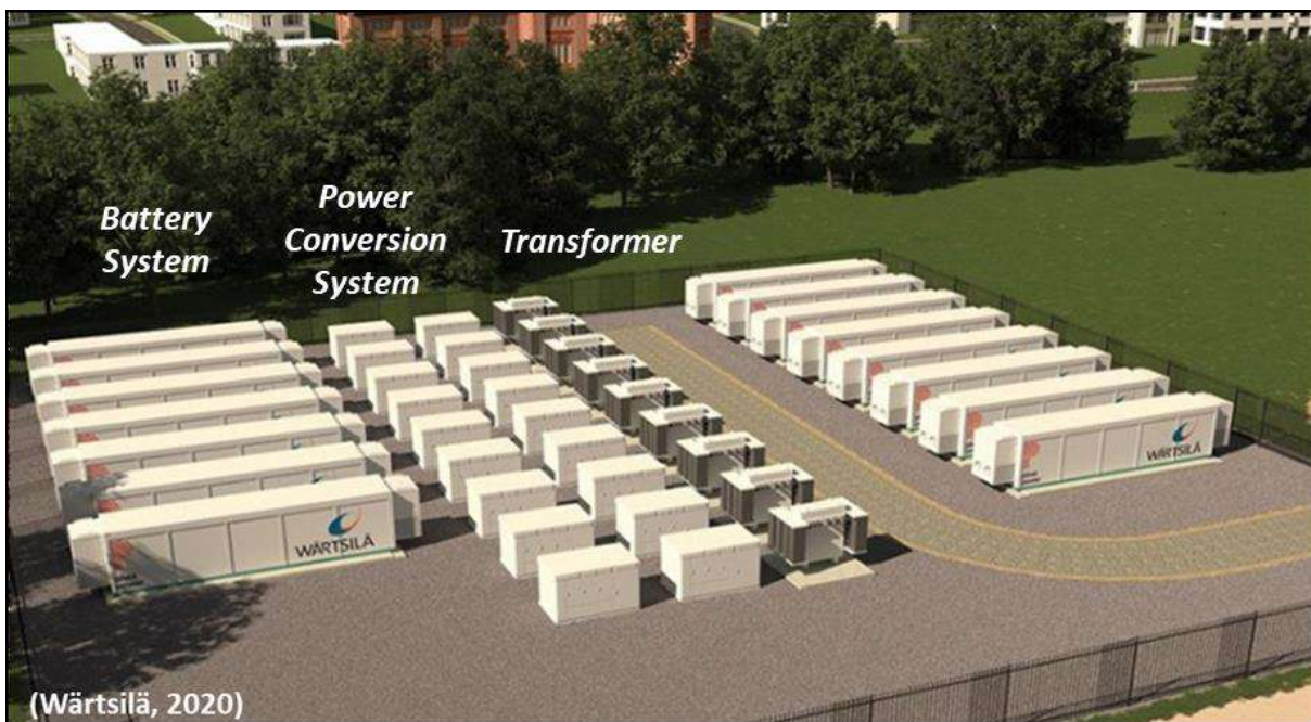
Figure 6: Example of a typical Battery Energy Storage System - Pivot Power's proposed lithium-ion battery in Kemsley, Kent.
