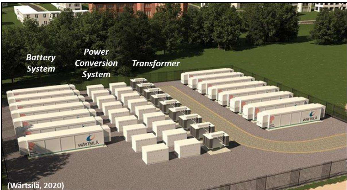
Figure 6: Example of a typical Battery Energy Storage System - Pivot Power's proposed 50MW lithium-ion battery in Kemsley, Kent.
