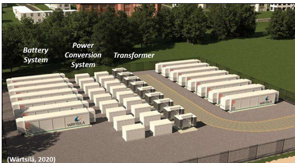
Figure 5: Example of a typical Battery Energy Storage System - Pivot Power's proposed 50MW lithium-ion battery in Kemsley, Kent.
