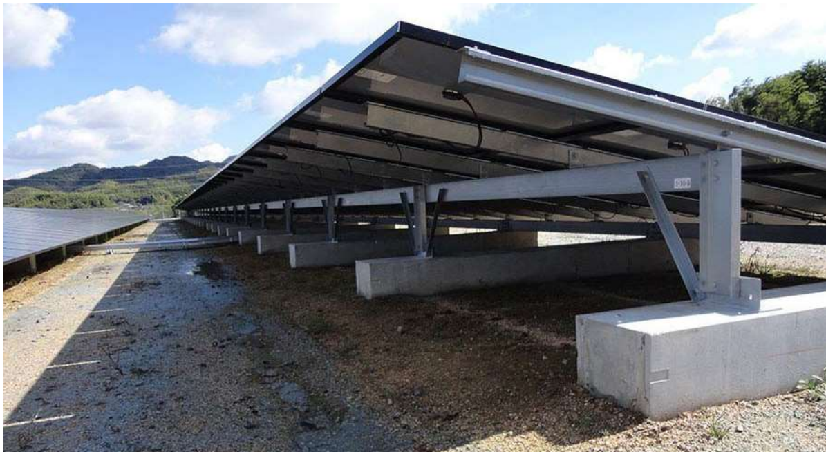
Figure 6: Cast Concrete Foundation (alternative mounting)
