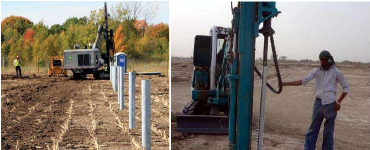
Figure 3: Driven/ Rammed Steel Pile (left) and Ground Screw (right) are the preferred mounting technology.
