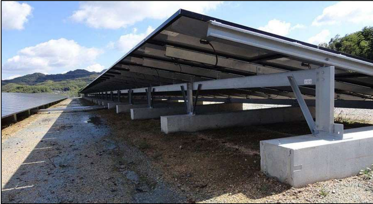
Figure 2: Cast Concrete Foundation (alternative mounting)
