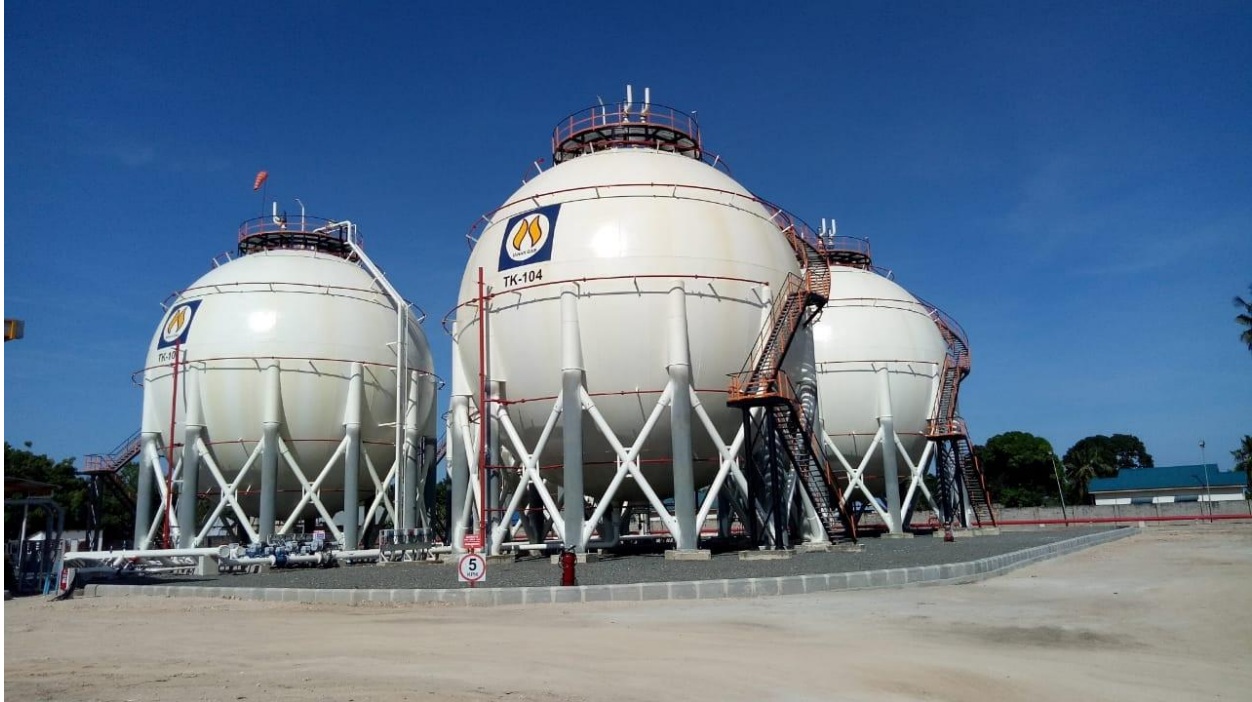
Figure 11: Sphere storage tanks
