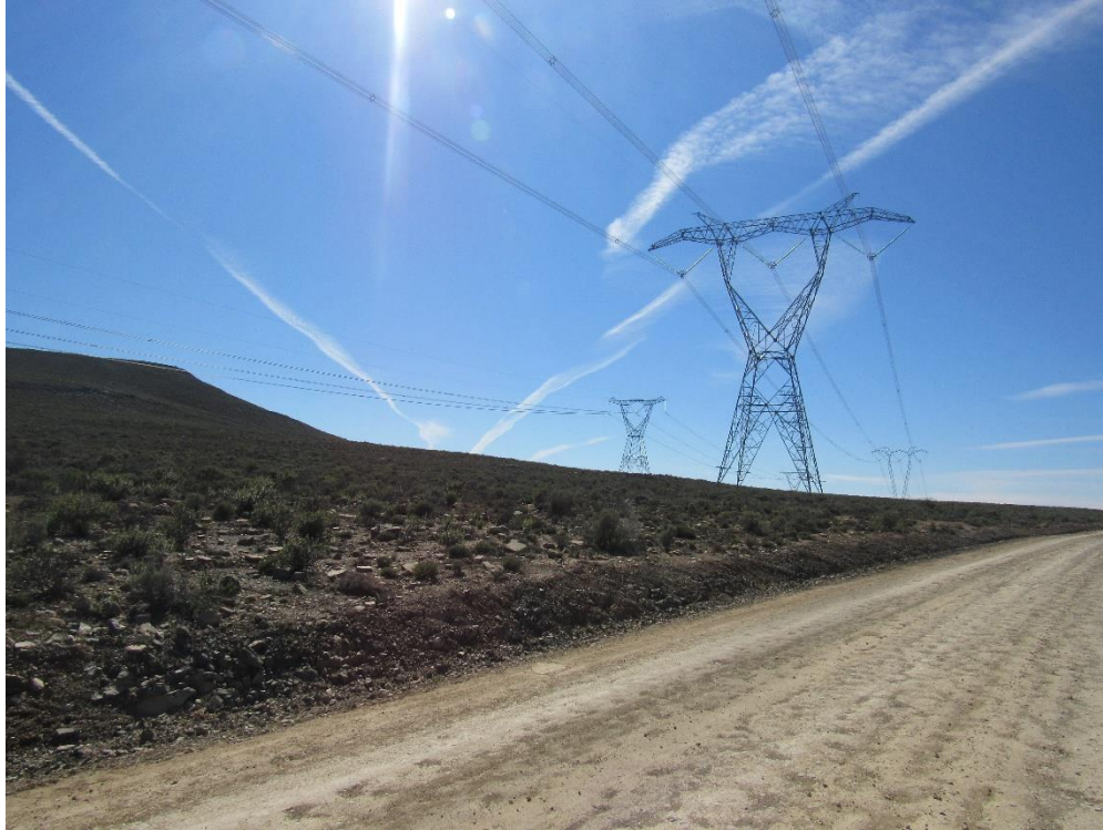
Figure 6-45: View of high voltage power lines in the study area
