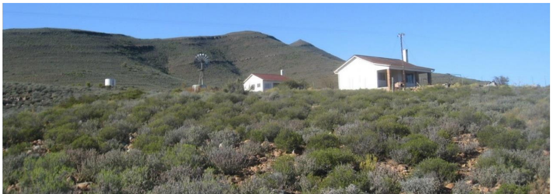
Figure 6-55: Caretaker staff accommodation (foreground) and farmstead on Klipbanks Fontein 198/1. The property forms part of an operation based in the Moordenaarskaroo
