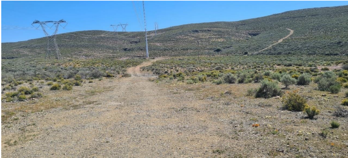
Figure 6-23: West of Substation Option 1
