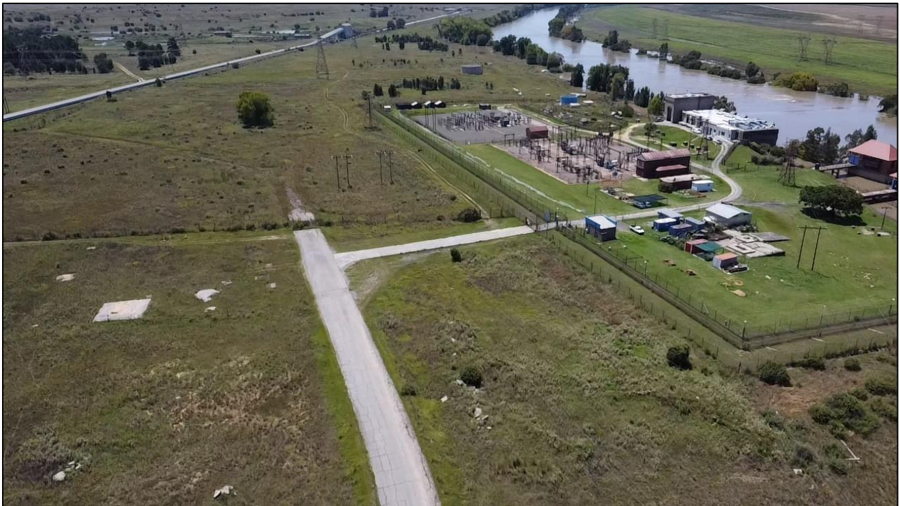
Figure 6-7: A view of the RWB substation
