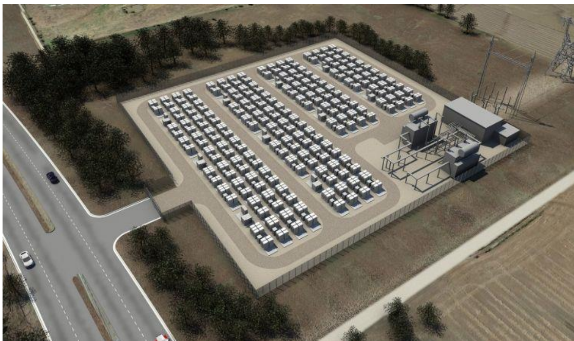
Plate 7-6: SolarCity's Tesla Battery Storage facility, Hawaii.
