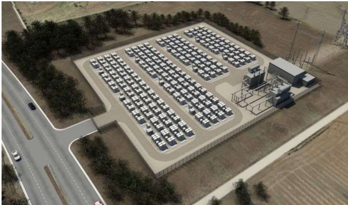
Plate 7-6: SolarCity's Tesla Battery Storage facility, Hawaii.
