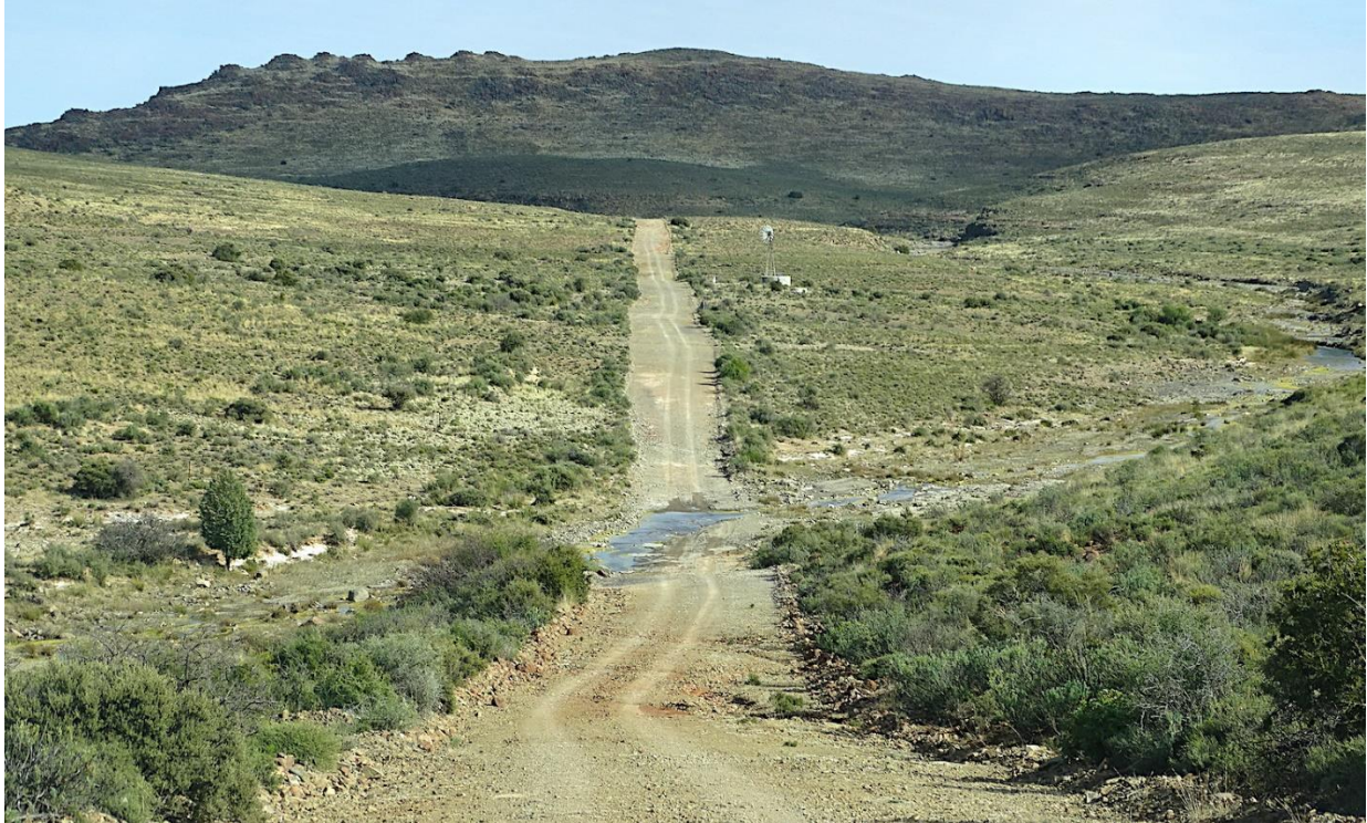
Figure 7-41 - Existing access road between Leeukloof and Booiskraal
