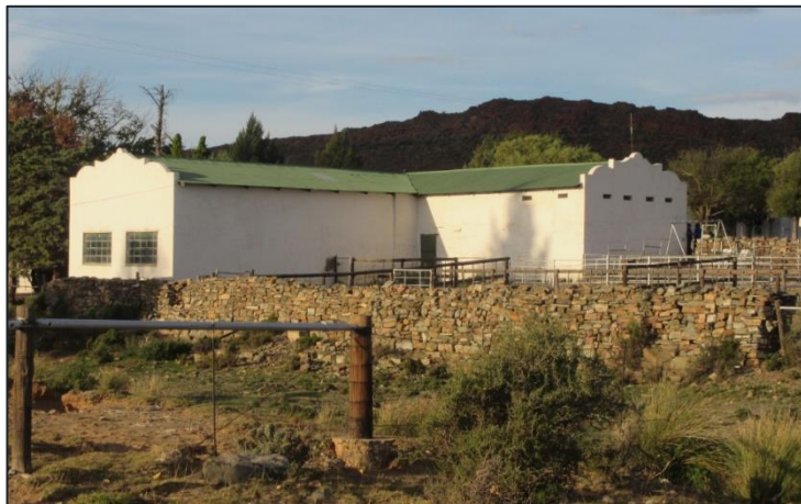
Figure 7-24 - Structure in the Leeukloof Farm complex at Waypoint 1850
