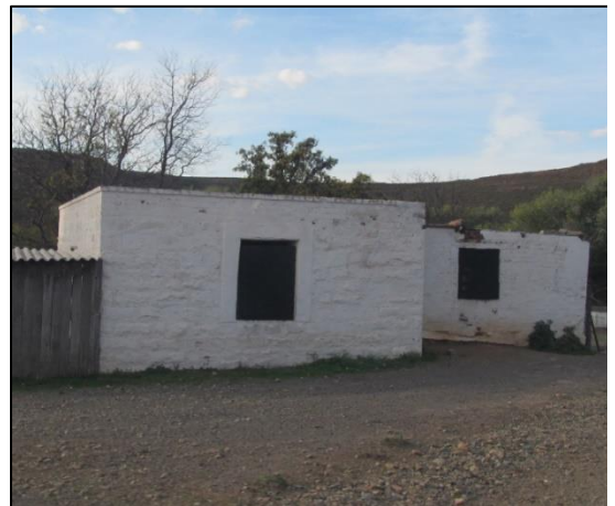
Figure 7-25 - Structure in the Leeukloof Farm complex at Waypoint 1850
