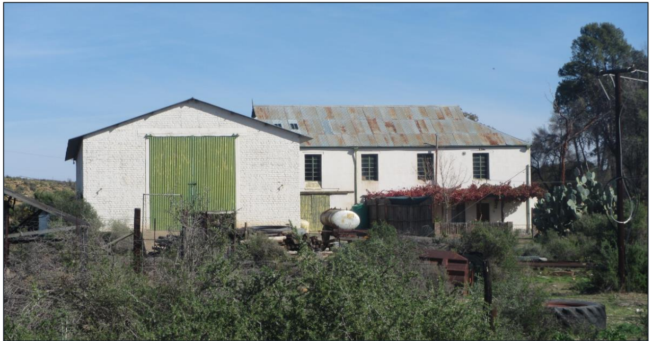
Figure 7-26 - A structure built of stone, sun-dried mud bricks and fired clay bricks at Waypoint 1993
