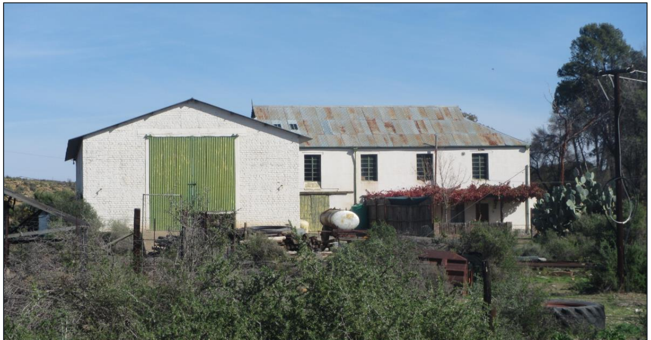
Figure 7-24 - A structure built of stone, sun-dried mud bricks and fired clay bricks at Waypoint 1993
