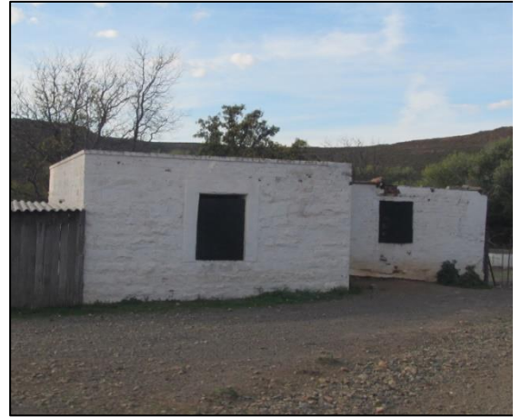
Figure 7-23 - Structure in the Leeukloof Farm complex at Waypoint 1850
