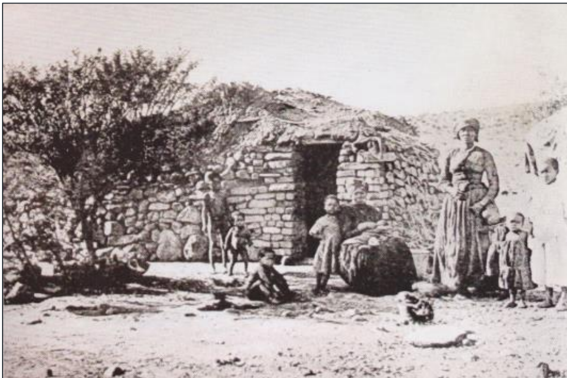
Figure 7-19 - A shepherd's hut photographed near Beaufort West in the early 20th century. Note the low, narrow doorway and informal roof structure. Source: Schoeman (2013:48)
