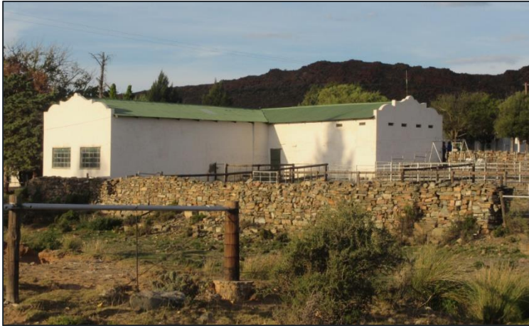
Figure 7-22 - Structure in the Leeukloof Farm complex at Waypoint 1850
