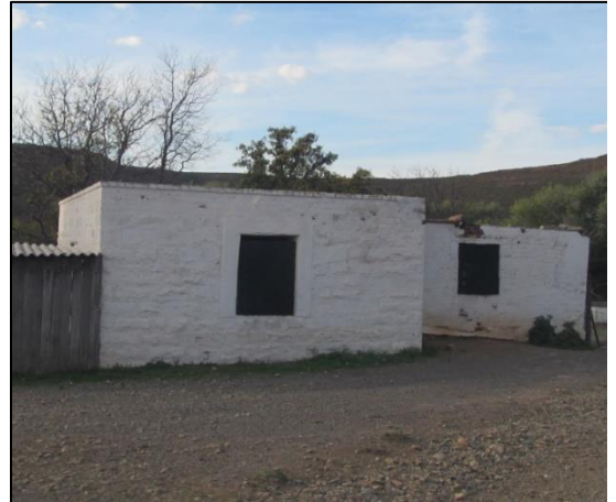
Figure 7-24 - Structure in the Leeukloof Farm complex at Waypoint 1850
