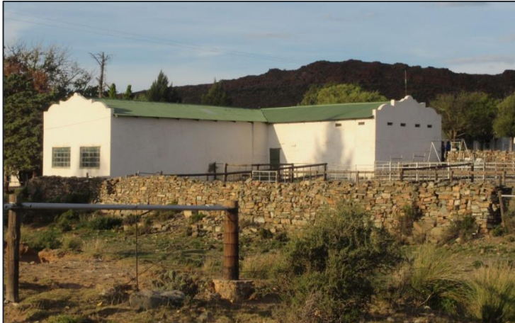
Figure 7-23 - Structure in the Leeukloof Farm complex at Waypoint 1850
