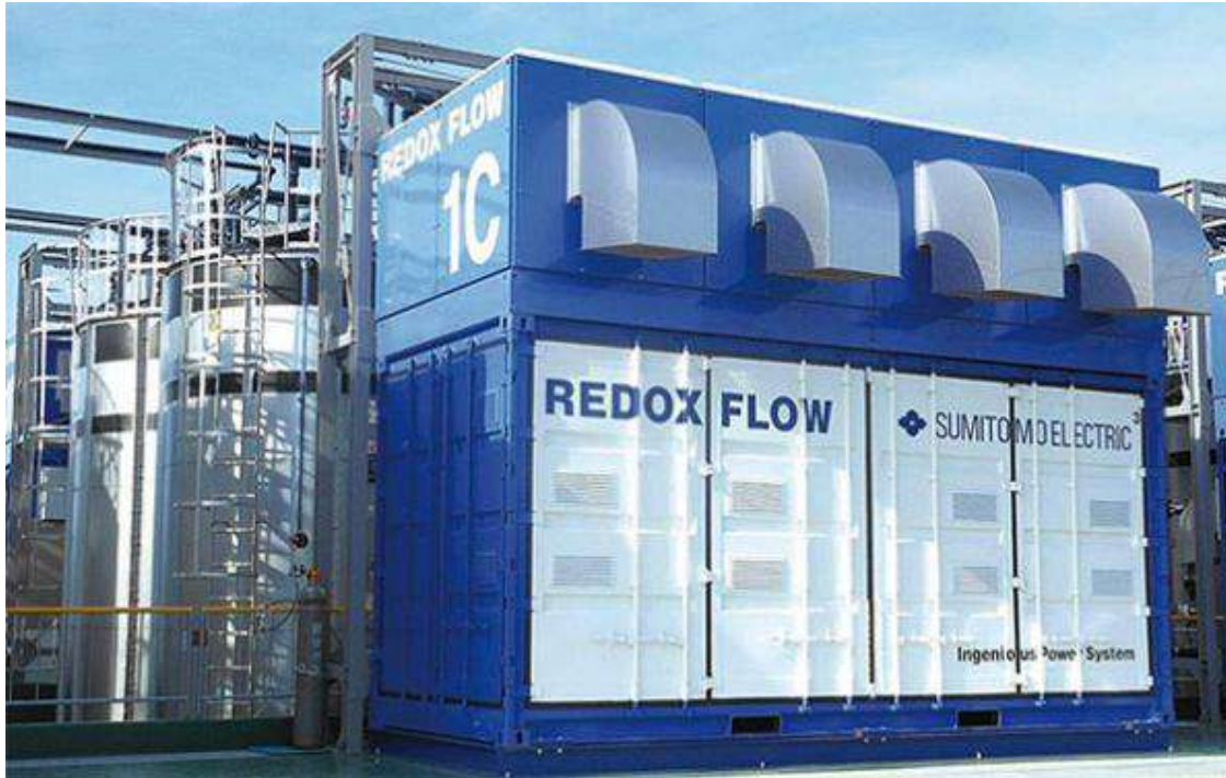
Figure 3-11 Standard BESS Design – VRF Flow Battery
