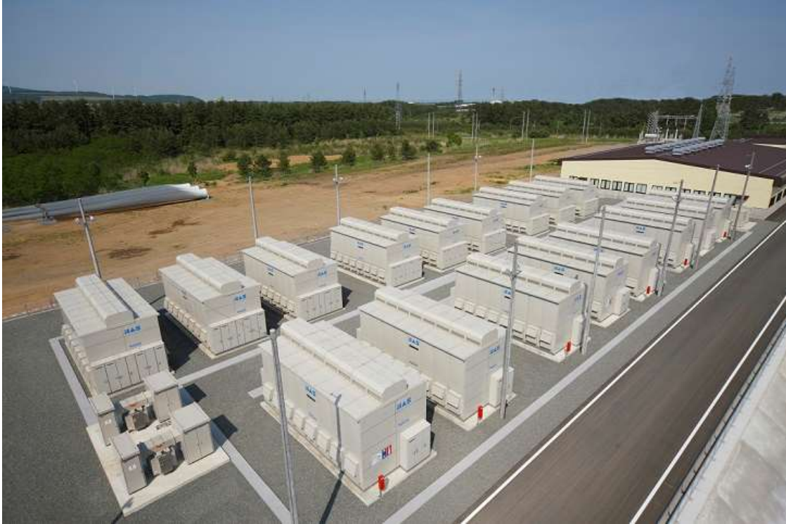
Figure 3-10 Standard BESS Design – NaS Solid State Battery
