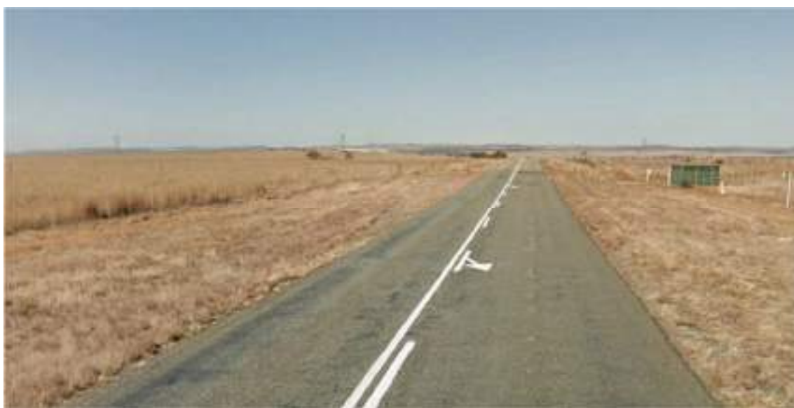
Figure 4-7: View in a southern direction on D331 at proposed access point
