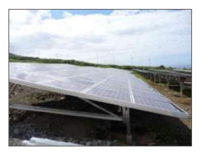
Figure 10: Fixed Solar PV Panels
