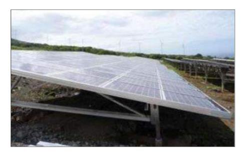
Figure 14: Example of Fixed Solar Panels (Nemai 2023)
