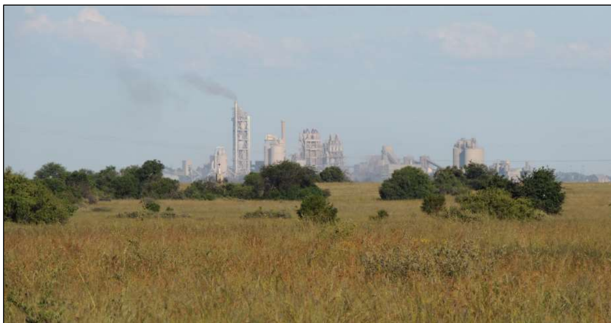
Figure 34. Photograph of the Lichtenburg LaFarge Cement Factory that forms a background view to much of the regional landscape (Stead, 2022)
