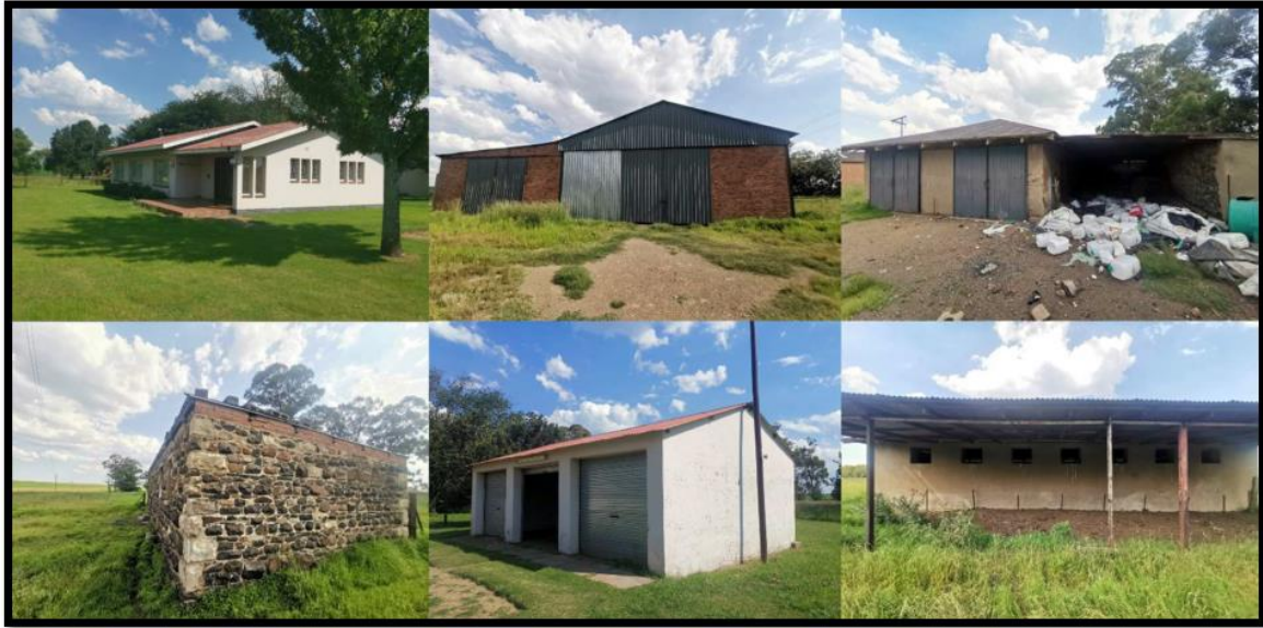
Figure 7-27 – Buildings that could act as potential bat roosts on the Project area of Influence
