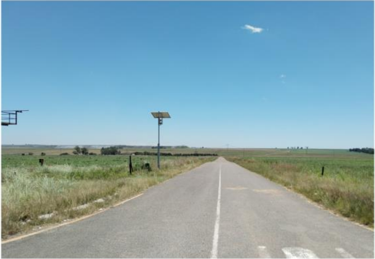
Figure 7-37 – Existing surfaced access road at Access point 1 towards the proposed site
