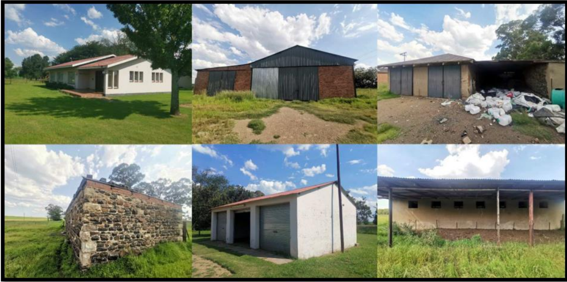
Figure 7-27 – Buildings that could act as potential bat roosts on the Project area of Influence
