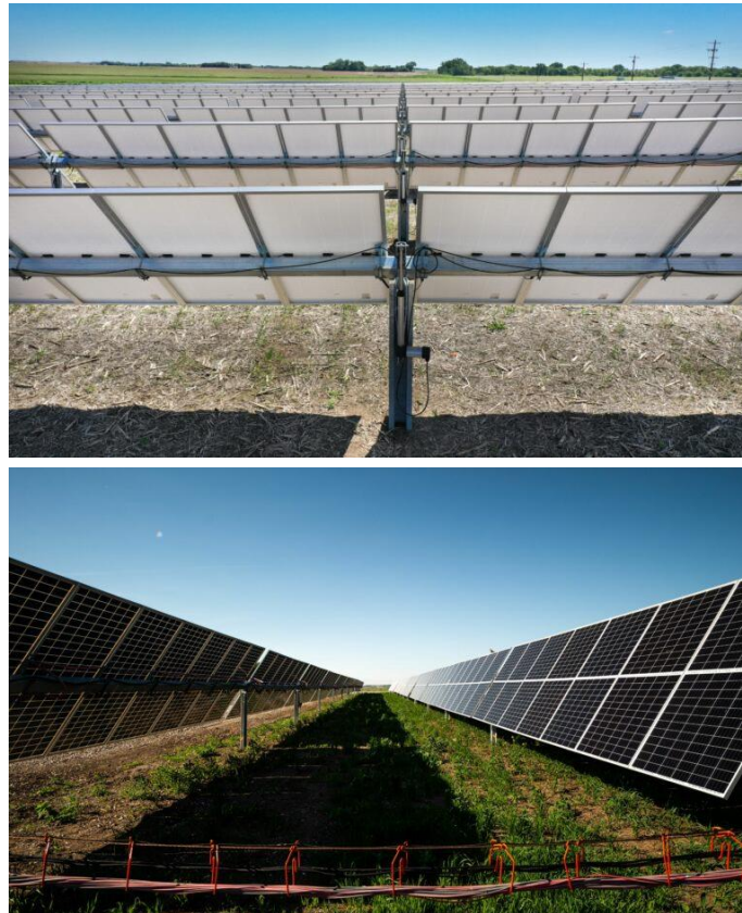
Figure 24: Monofacial (top) and bifacial (bottom) solar panels
