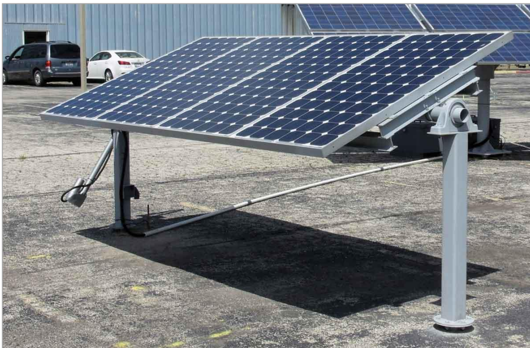
Figure 12: Example of PV Module mounted on Single Axis Tracker (source: Single-ACES – Atlantic Clean Energy Supply – Official Site [ https://atlanticces.com/ ])
