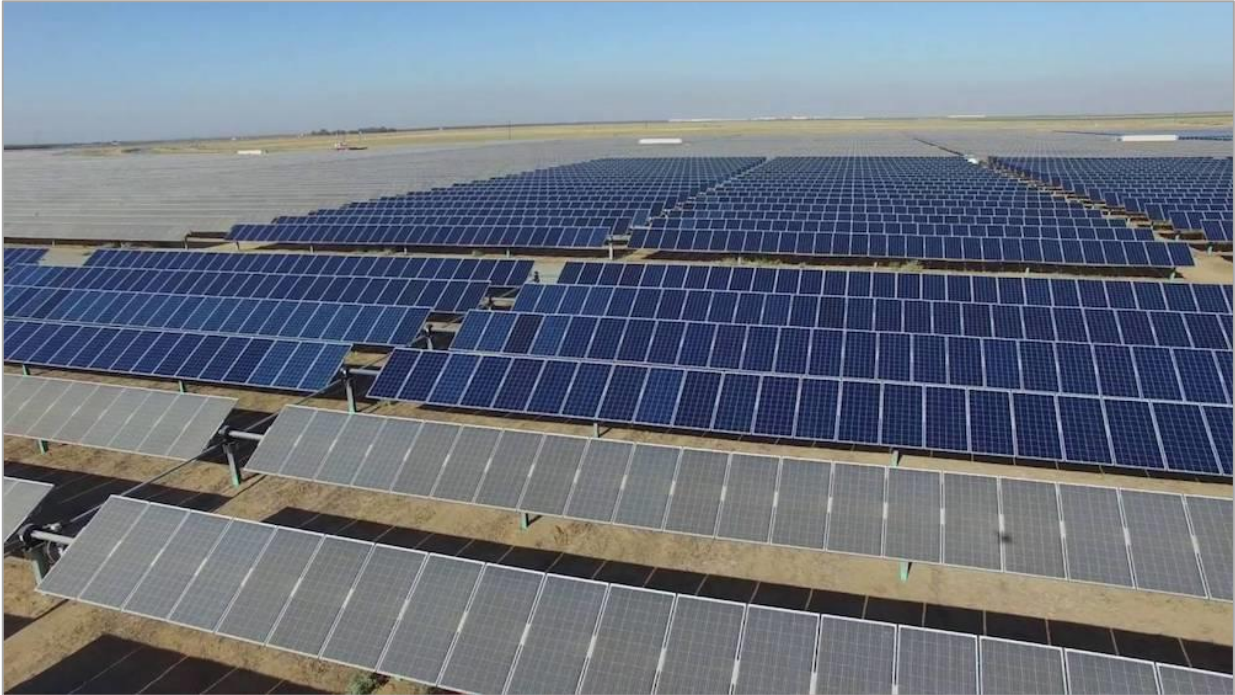
Figure 16: Example of Roads Between Trackers and Medium Voltage Substations (source: https://ecoinventos.com/ )
