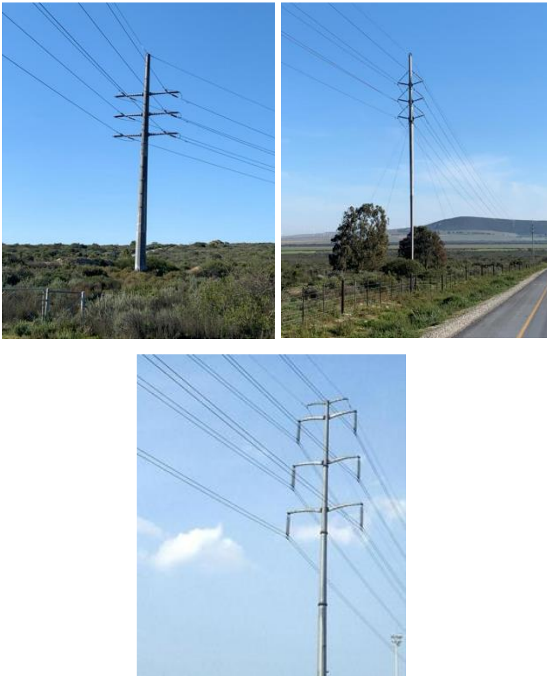
Plate 4-1: Proposed Self-supporting Steel / Concrete Monopoles.
