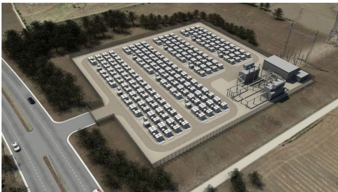
Plate 3-1: SolarCity's Tesla Battery Storage Facility, Hawaii. [Source: https://www.pv-tech.org/news/solarcity-picks-tesla-for-52mwh-of-dispatchable-solar-plus-storage-in-hawaii ]
