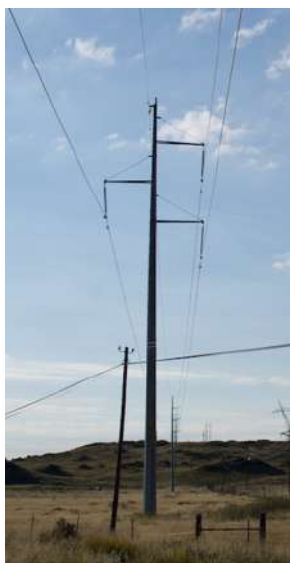
Figure 4-1: Example of a Self-supporting Monopole.
