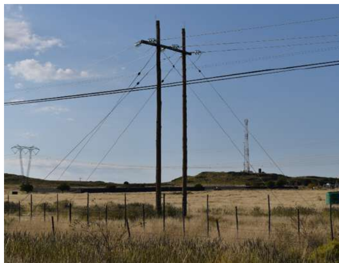
Figure 4-2: Example of a Guyed-suspension.
