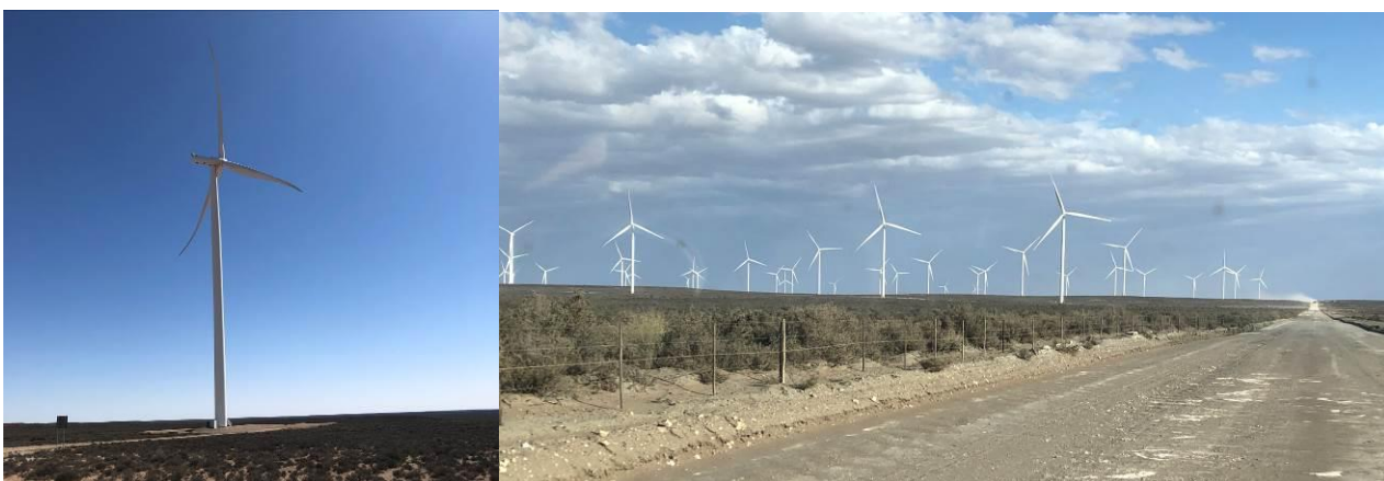
Figure 2-4: Example of an operational wind farm.
