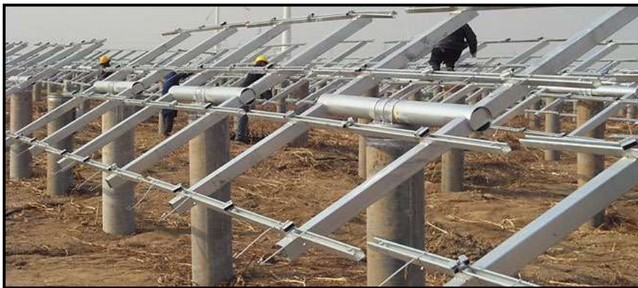
Figure 13 Support structure for Tracking PV Panels
