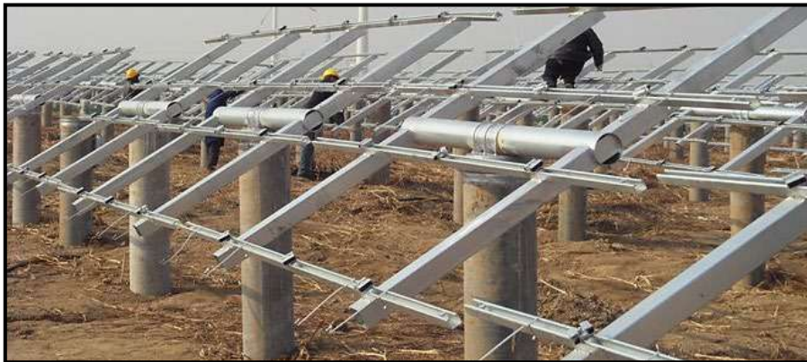
Figure 13 Support structure for Tracking PV Panels
