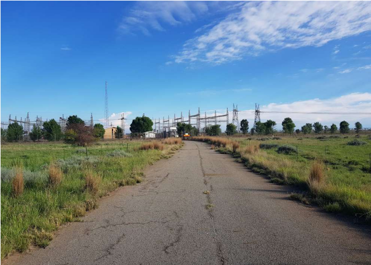
Figure 45: Existing Eskom Substation
