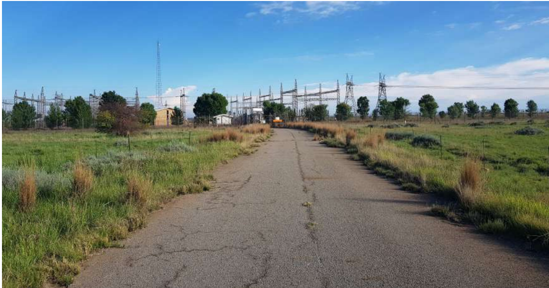
Figure 27: Existing Eskom substation as viewed from the R76 looking north.
