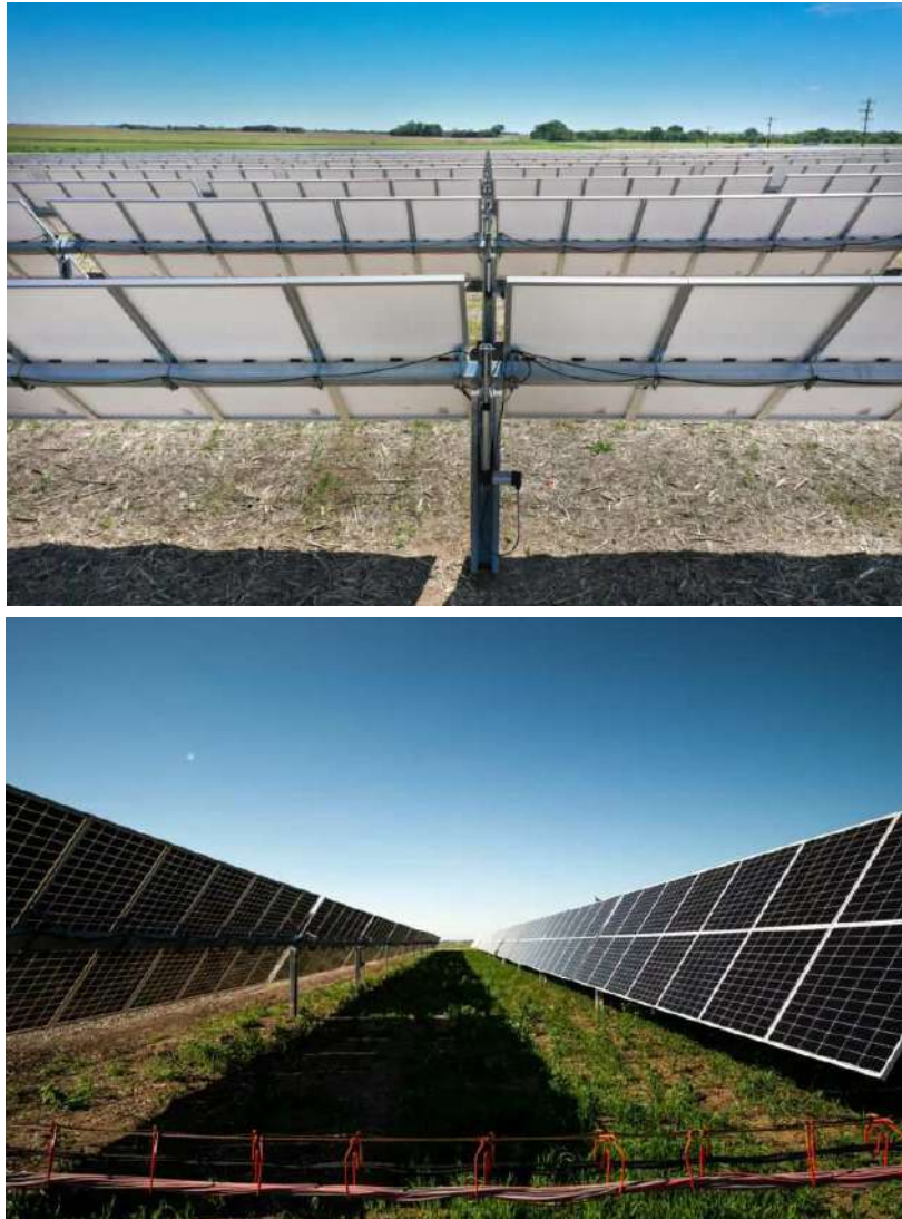
Figure 26: Monofacial (top) and bifacial (bottom) solar panels (
