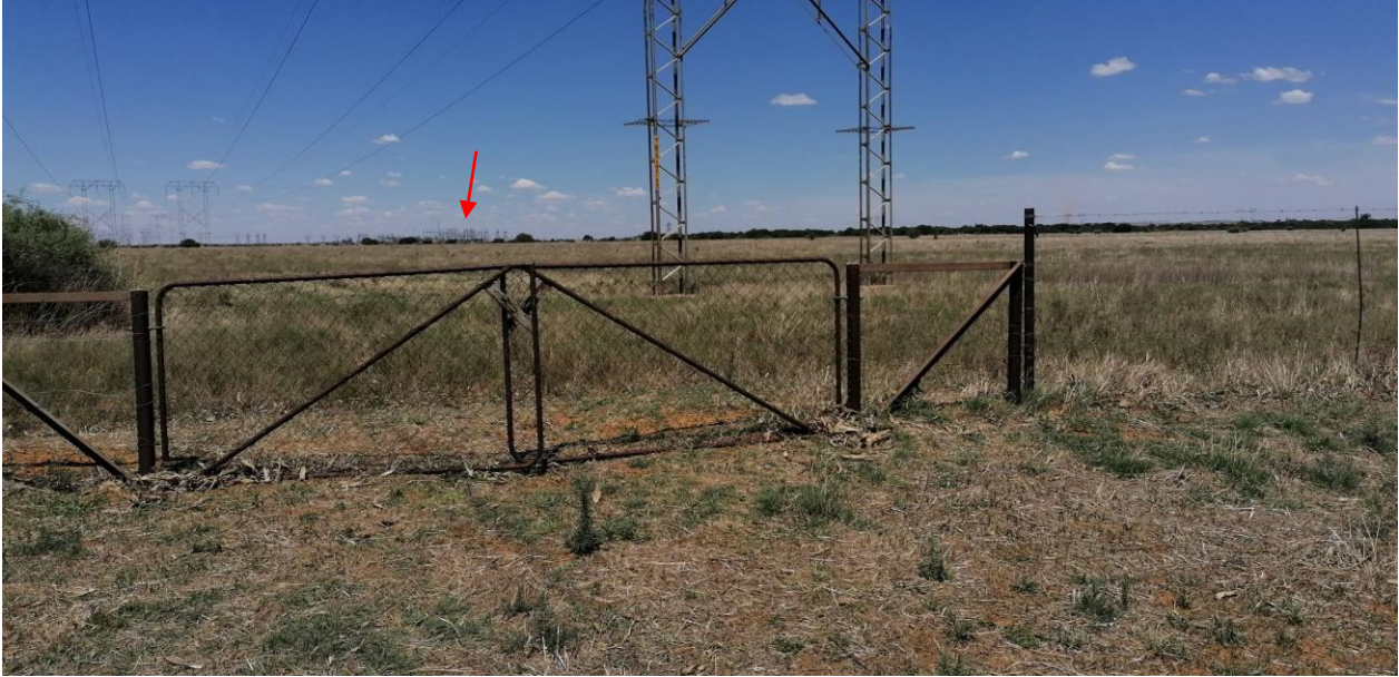
Figure 5: General view of part of the proposed site looking east. The existing powerlines can be seen, as well as the Theseus Substation in the distance (red arrow).
