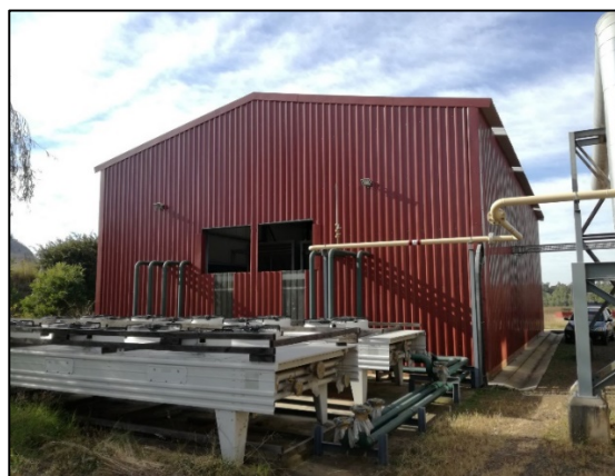
Figure 6-1 (c): Powerhouse containing Jenbacher engines
