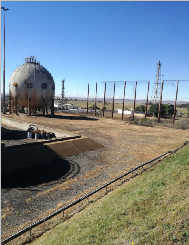
Figure 6-7 (c): View of proposed LNG Tank Farm area
