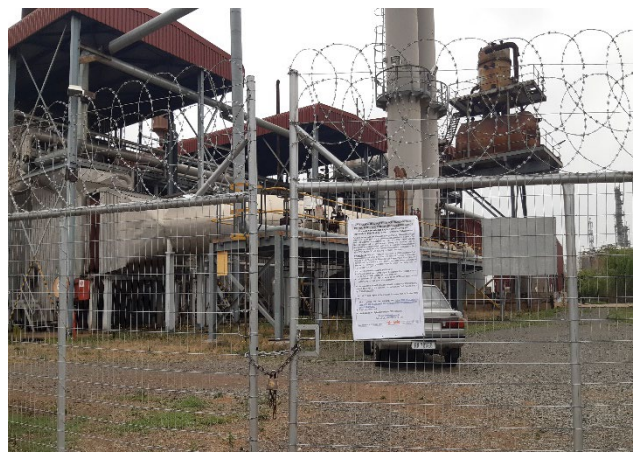
Plate 4: Site Notice placed at Newcastle Energy Main Entrance (27°47'8.22"S; 29°58'8.95"E)
