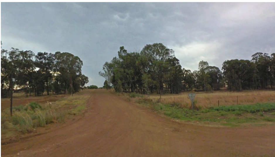
Figure 6.2: Gravel access road from the R505 arterial road
