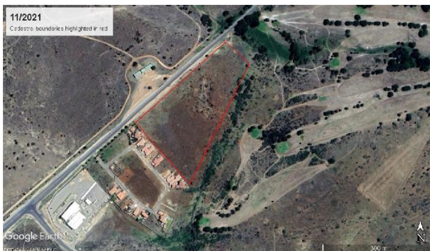
2021 Google Earth aerial image
