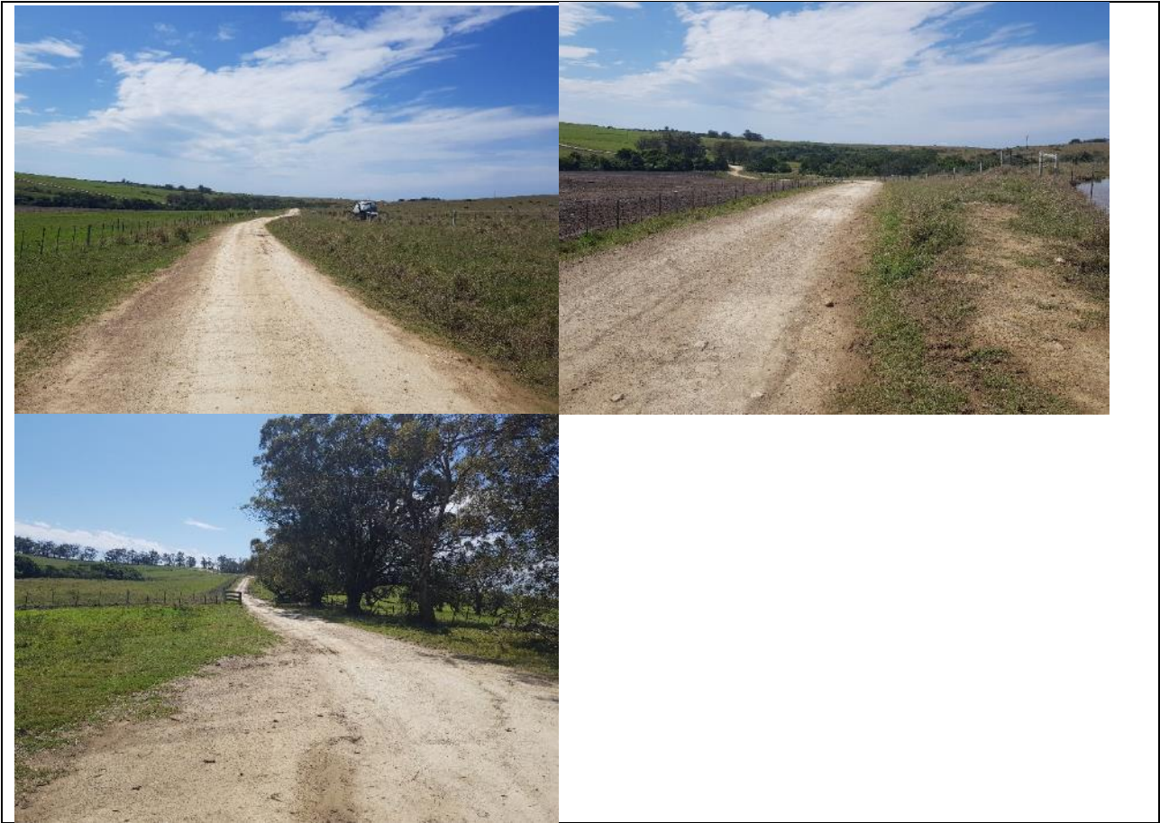
Plate A: Site Photographs: Section 1 & 2
