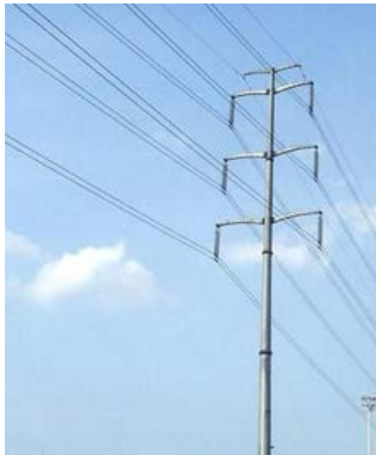
Plate 4-1: Proposed Self-supporting Steel / Concrete Monopoles.
