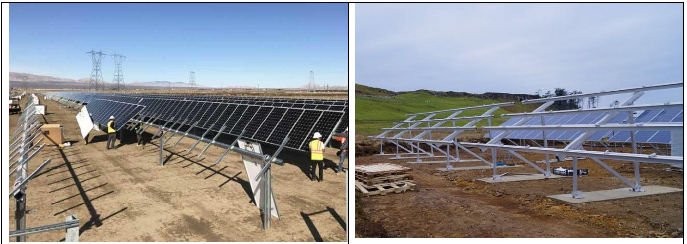
Figure 2.7: Photographs illustrating frame structural details
