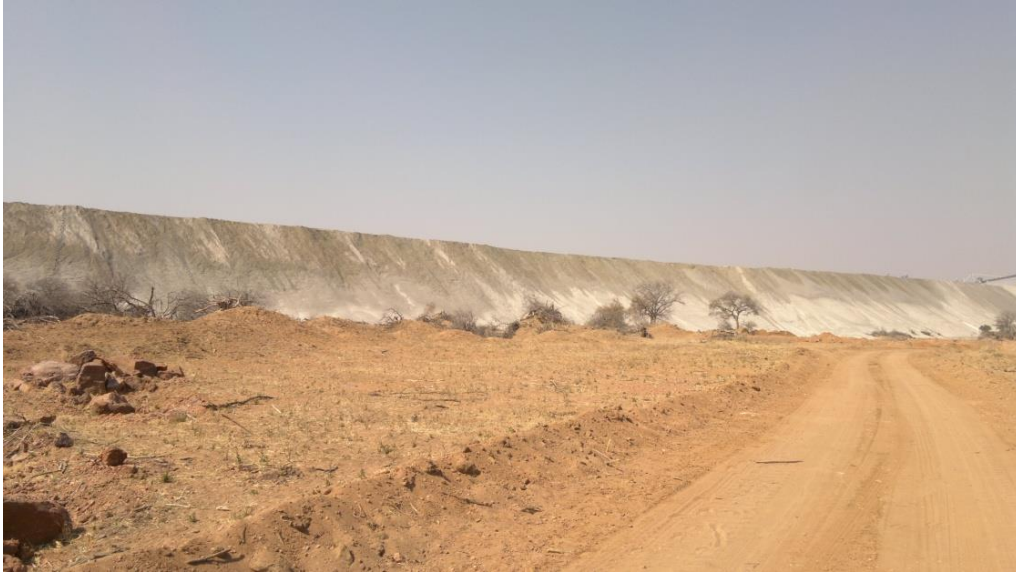
Figure 11: Advancing face of existing ash facility
