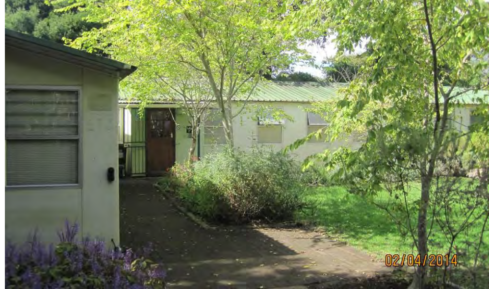
Prefabricated structures to be demolished.
