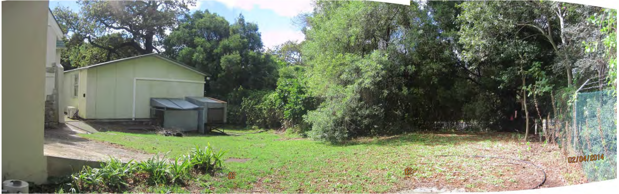
The southern end of the prefabricated structure and the relationship between the site and Rhodes Drive – Rhodes rive can just be seen through the vegetation and fence on the right hand side of the photograph. The corner of Fynbos Lodge can be seen on the left in the background (with stone rustication) and another modern outbuilding (to be retained) is on the left in the foreground.
