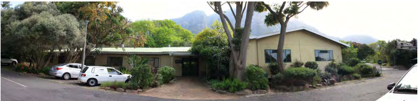
Photo Plate 4 – Existing prefab building, which will be replaced by a 2.5 storey Administration building
