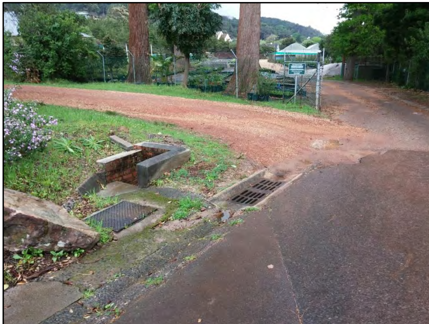
Figure 1: Typical Example of existing stormwater infrastructure.
