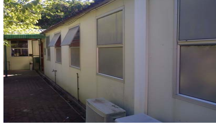
Figure 2: North view of the existing single story prefabricated IT building.
