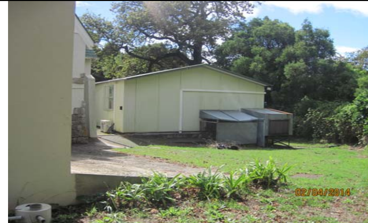
Figure 6: North-east view of the back of the Fynbos Lodge (left) and the prefabricated IT building (centre)
