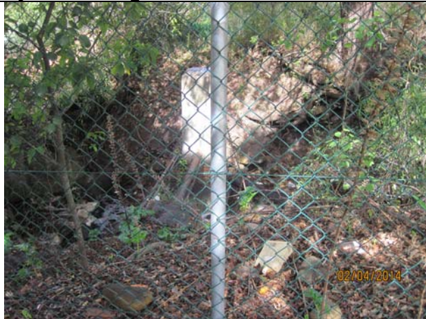
Figure 11: South-East view of the concrete culvert related infrastructure
