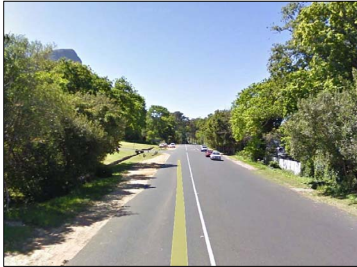
Photo 1: Northbound view along Rhodes Drive
