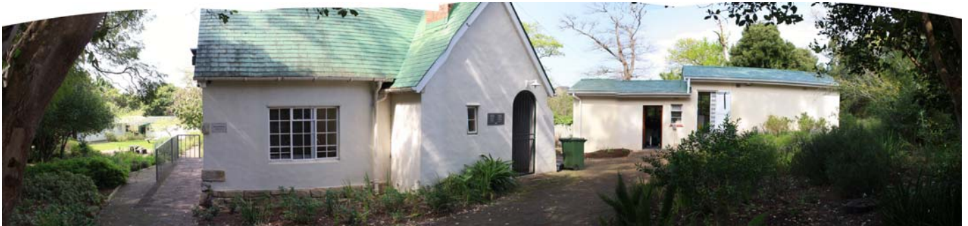
Photo Plate 7 – The existing Fynbos lodge building, left, which has heritage significance and the outbuildings, all of which will be retained.
