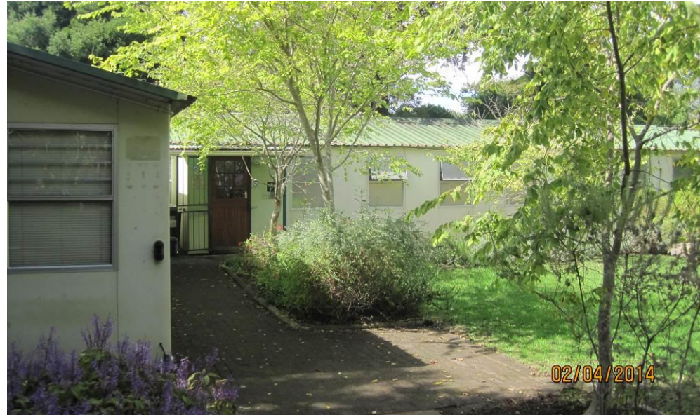
Prefabricated structures to be demolished.
