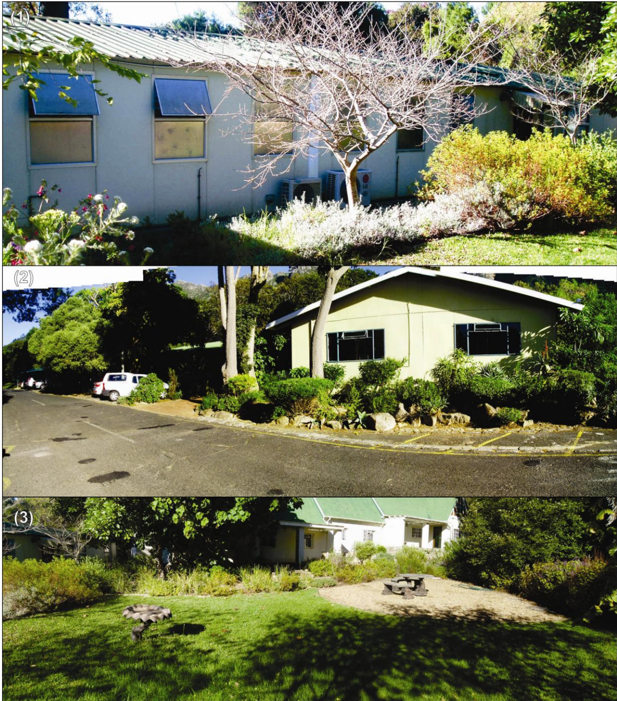
Figure 7 Existing administrative infrastructure in Kirstenbosch NBG: (1) IT Building, (2) Administration Building showing the existing parking lot and (3) the 'Fynbos Lodge'
