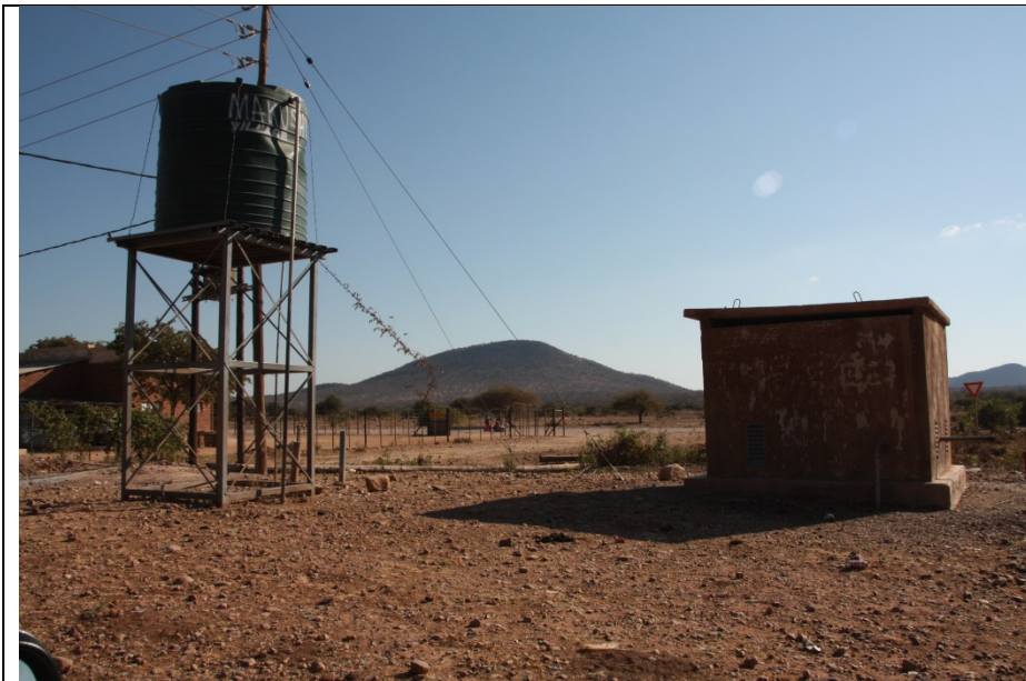
Borehole and watertank
