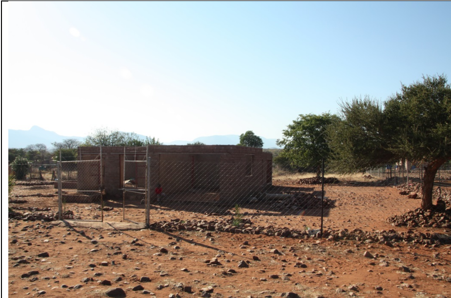
Brick and mortar house being build
