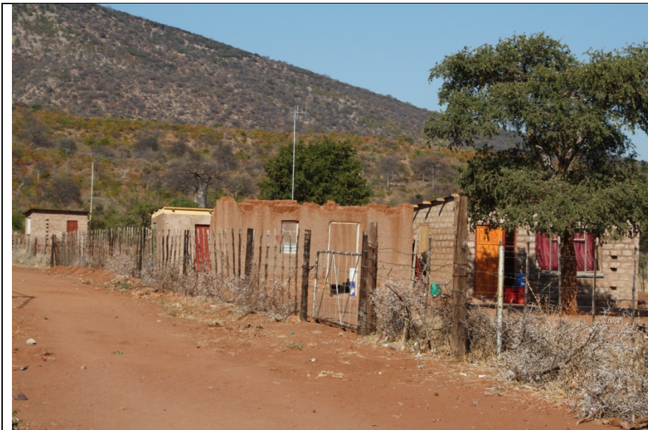
Old mud house with newer structures
