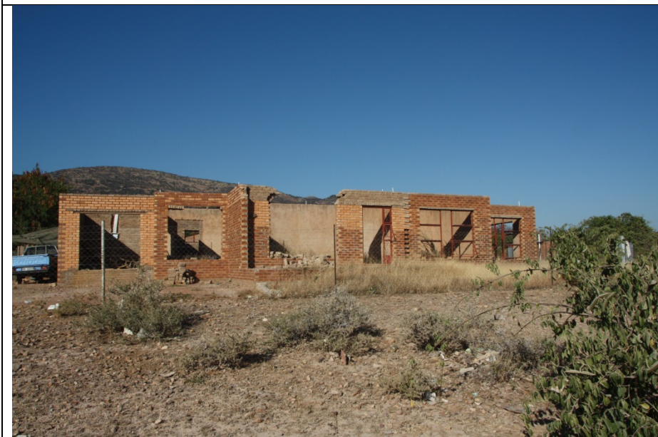
House being built
