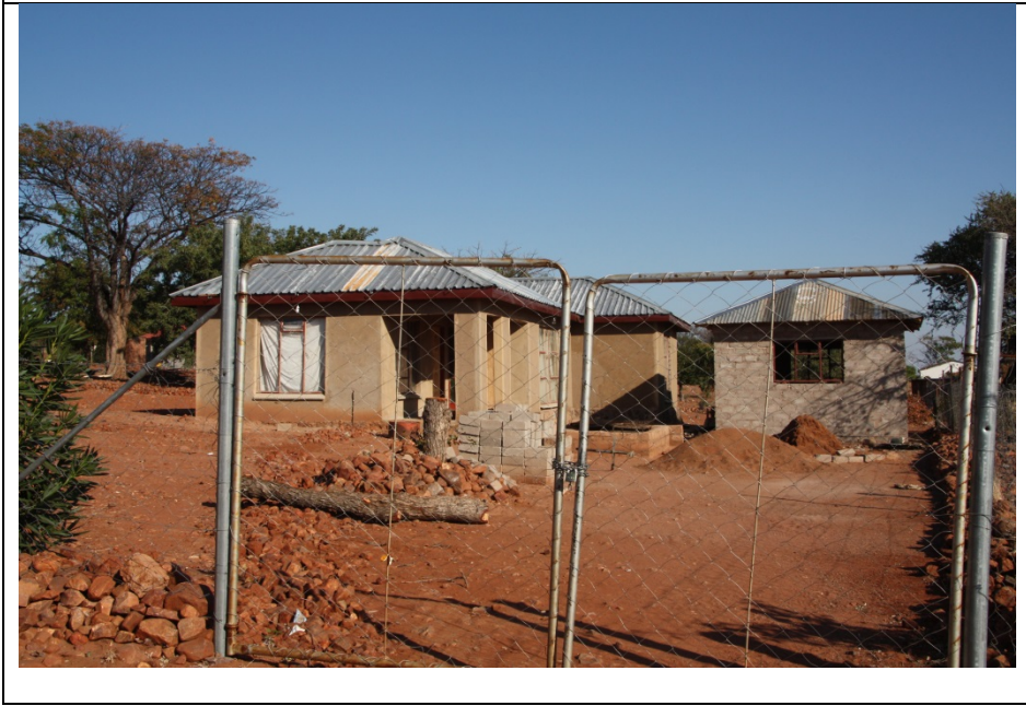
Relatively new structure
