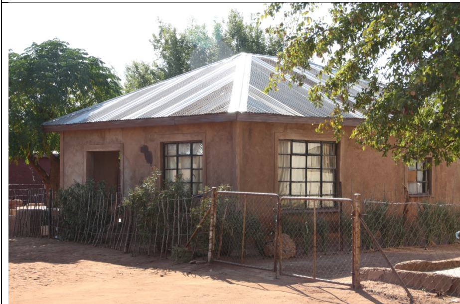
House with corrugated iron roof
