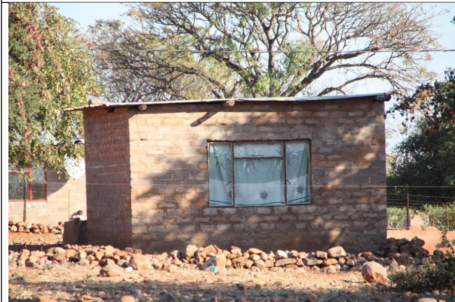
Brick and mortar house and corrugated iron roof
