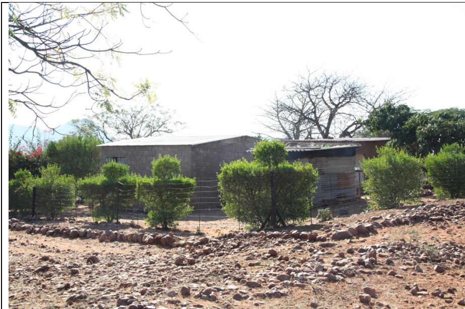
Cement brick and mortar house
