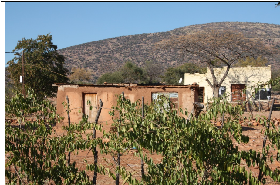
Old structure build with mud walls
