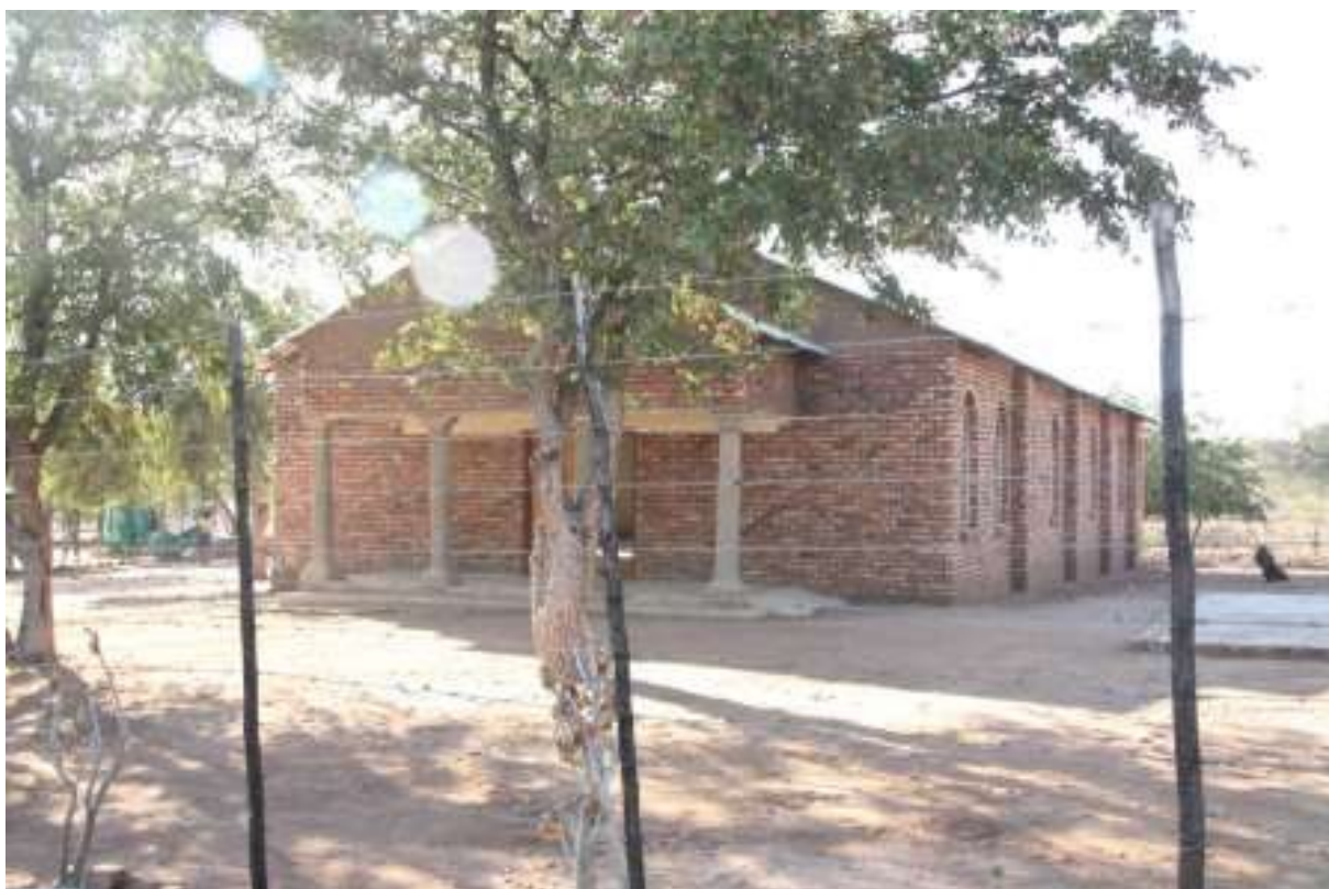
Figure 25: Church building located in Mosholombe
