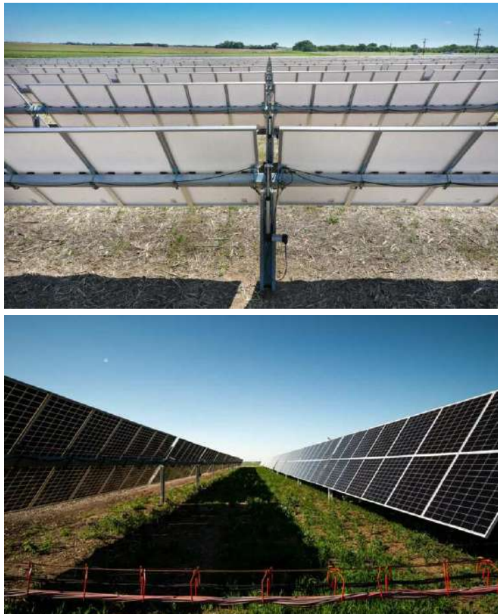
Figure 21: Monofacial (top) and bifacial (bottom) solar panels
