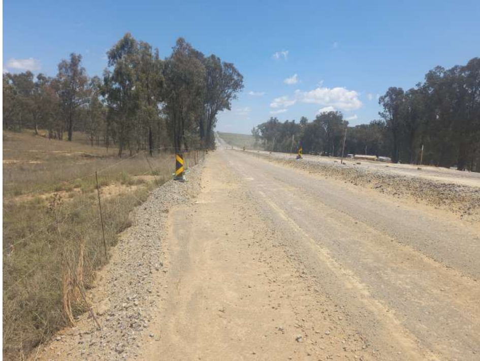
Figure 42: Upgrade of the R76 (PV Site on left-hand side)
