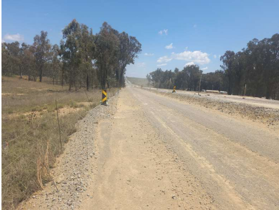
Figure 45: Upgrade of the R76 (PV Site on left-hand side)
