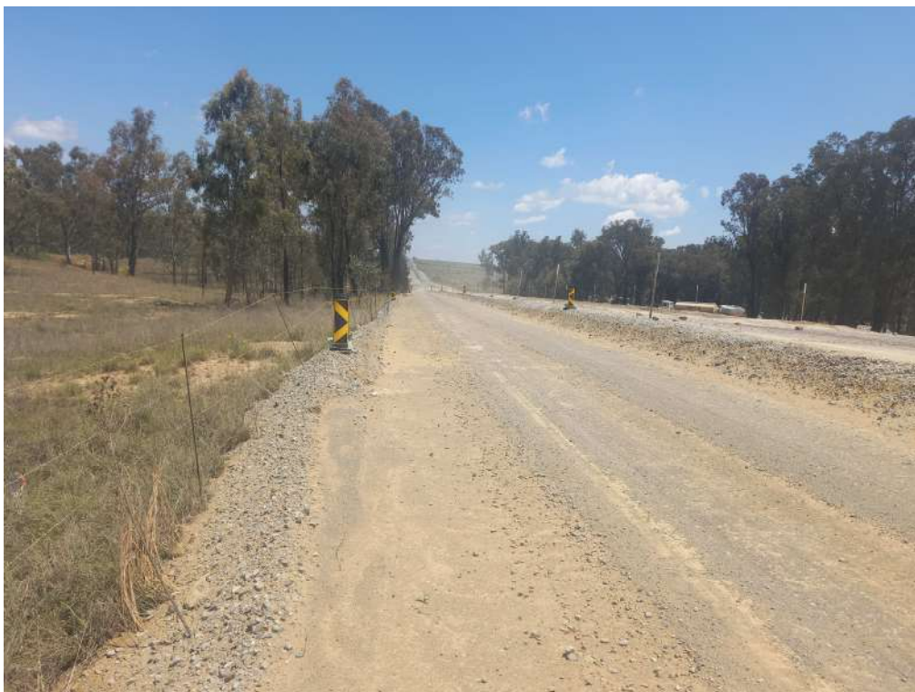
Figure 25: Construction along the R76
