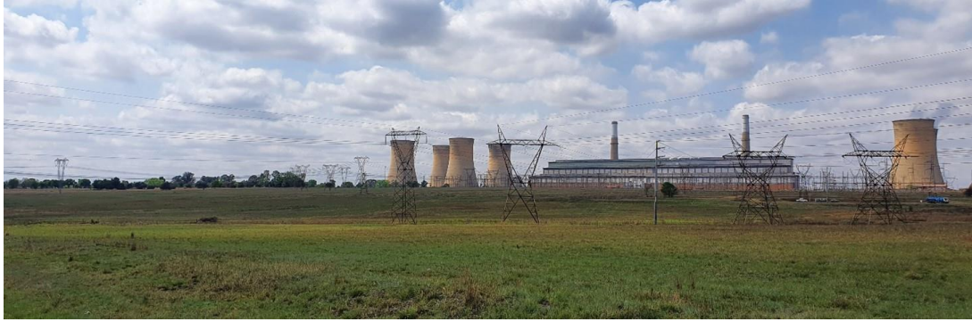
Figure 5: Power plant, and power lines traversing the landscape
