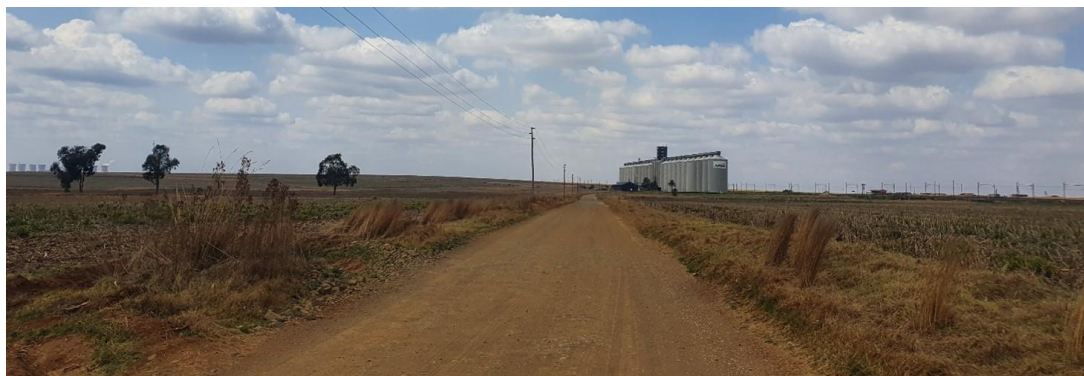
Figure 7: Afgri grain silo
